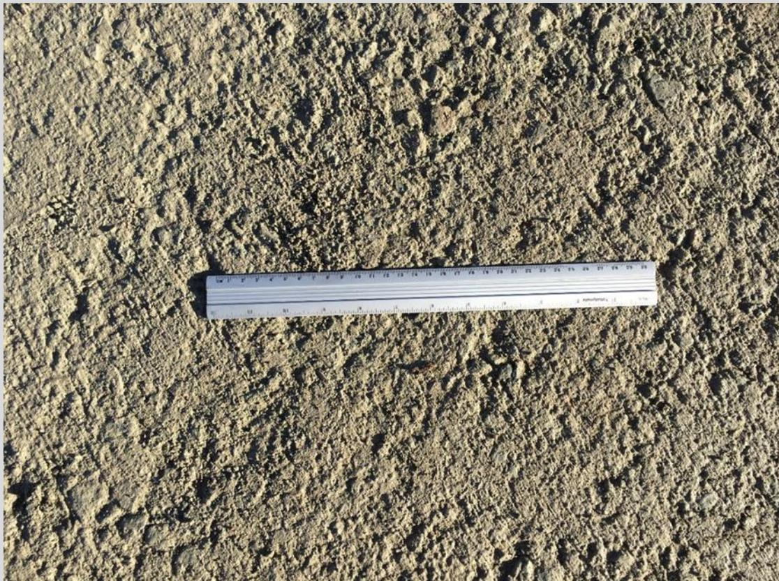
Unless the overlying layer is being constructed in the same work shift, a cement slurry (refer Clause 6.4) shall be applied to the hard-cut surface prior to placing the next heavily bound pavement layer.
