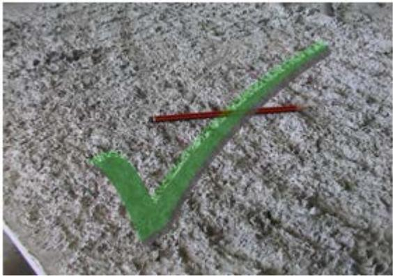
**Figure 7 Not acceptable, too rough not holding aggregate in place**
