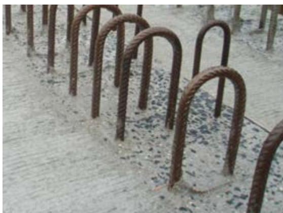
**Figure 2 Required finish under case in-situ kerb**
