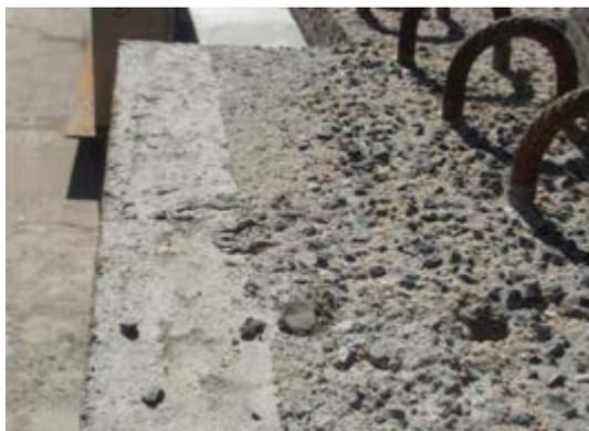
**Figure 5 Required finish on girders**
