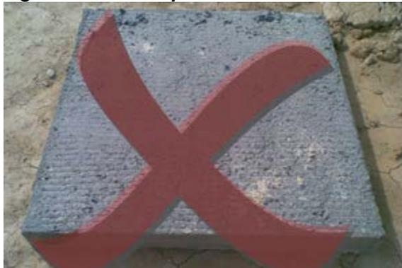
**Figure 11 Not acceptable rake finish**
