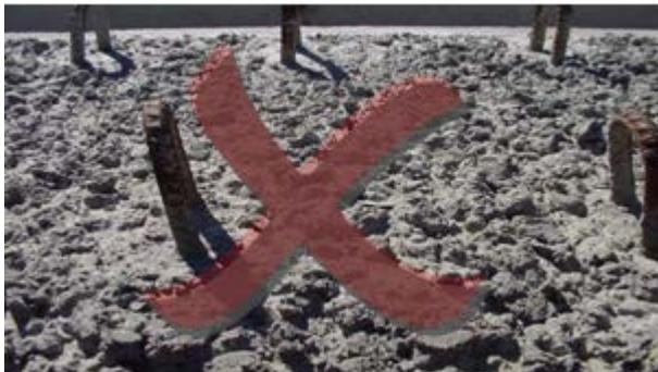
**Figure 8 Not acceptable, concrete laitance to be avoided, surface too smooth**
