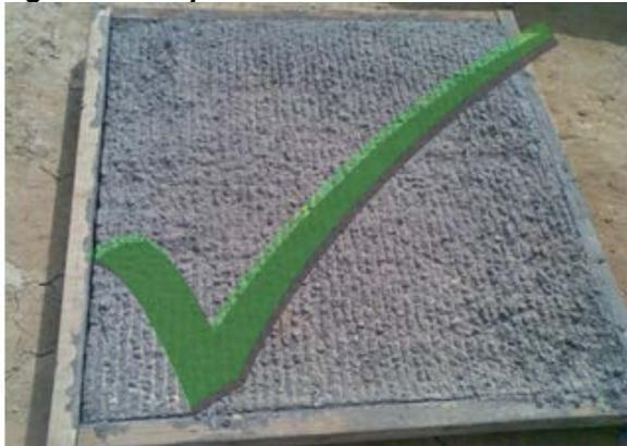
**Figure 10 Not acceptable rake finish**
