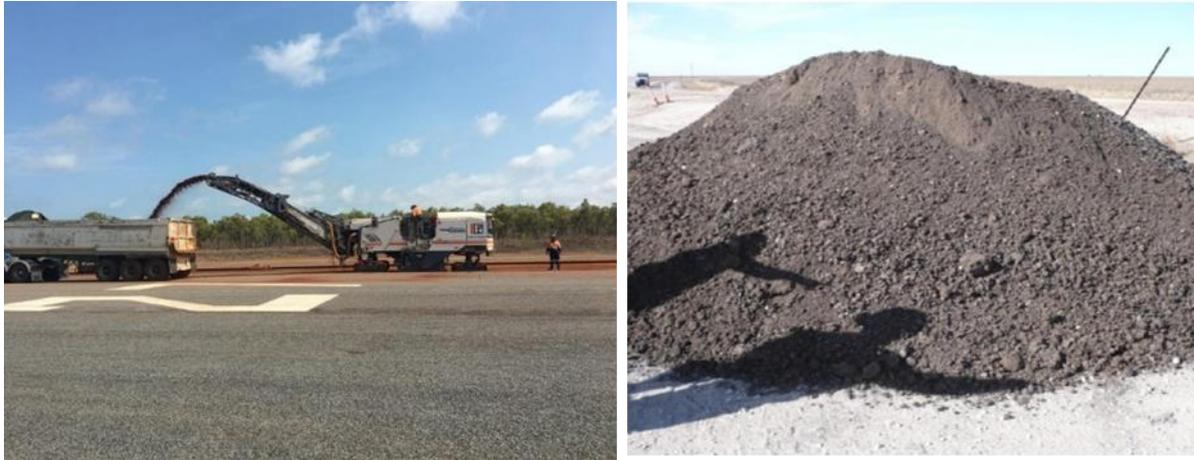
Current Transport and Main Roads specifications allow the incorporation of RAP into dense graded asphalt mixes for surfacing, intermediate, base and corrector courses. [MRT30 Asphalt Pavements](#), [MRTS32 High Modulus Asphalt \(EME2\)](#) and [MRTS102 Reclaimed Asphalt Pavement Material](#) set out the requirements for RAP that is used in asphalt.
