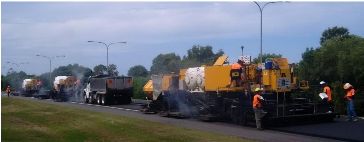
Currently, the department does not have a standard specification for HIPAR. Transport and Main Roads' [Pavement Rehabilitation Manual](#) (Section 4.4.14) provides guidance on the use of HIPAR including the required materials and design considerations.
