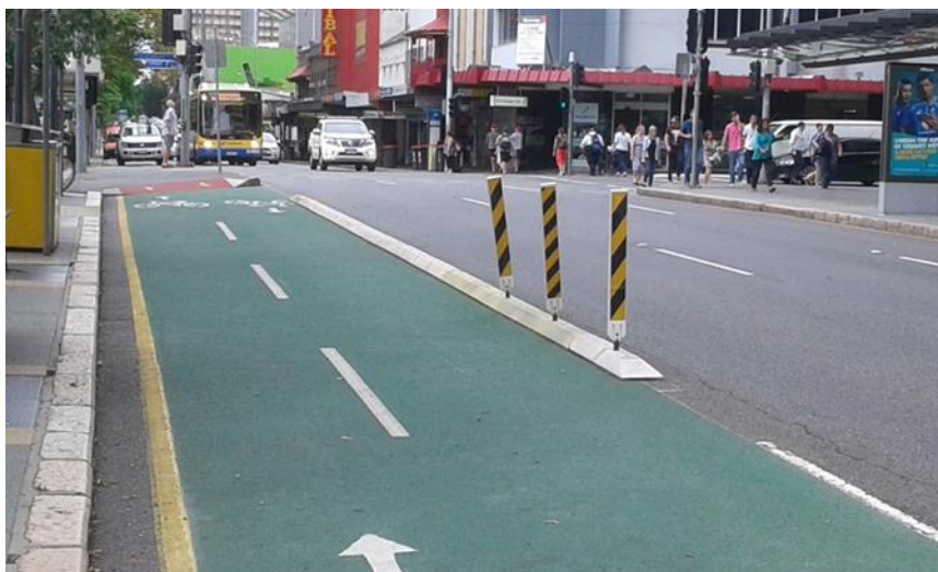
Figure 4.1.2(B) – George Street, Brisbane (plastic kerb with vertical delineators)
