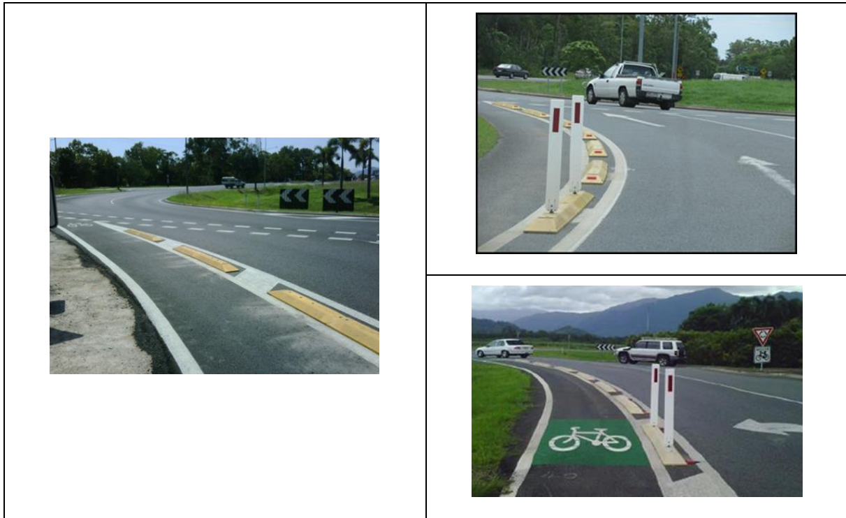
Figure 4.1.2(A) – Captain Cook Highway: 2009 separation treatment (plastic kerb with vertical delineators)
