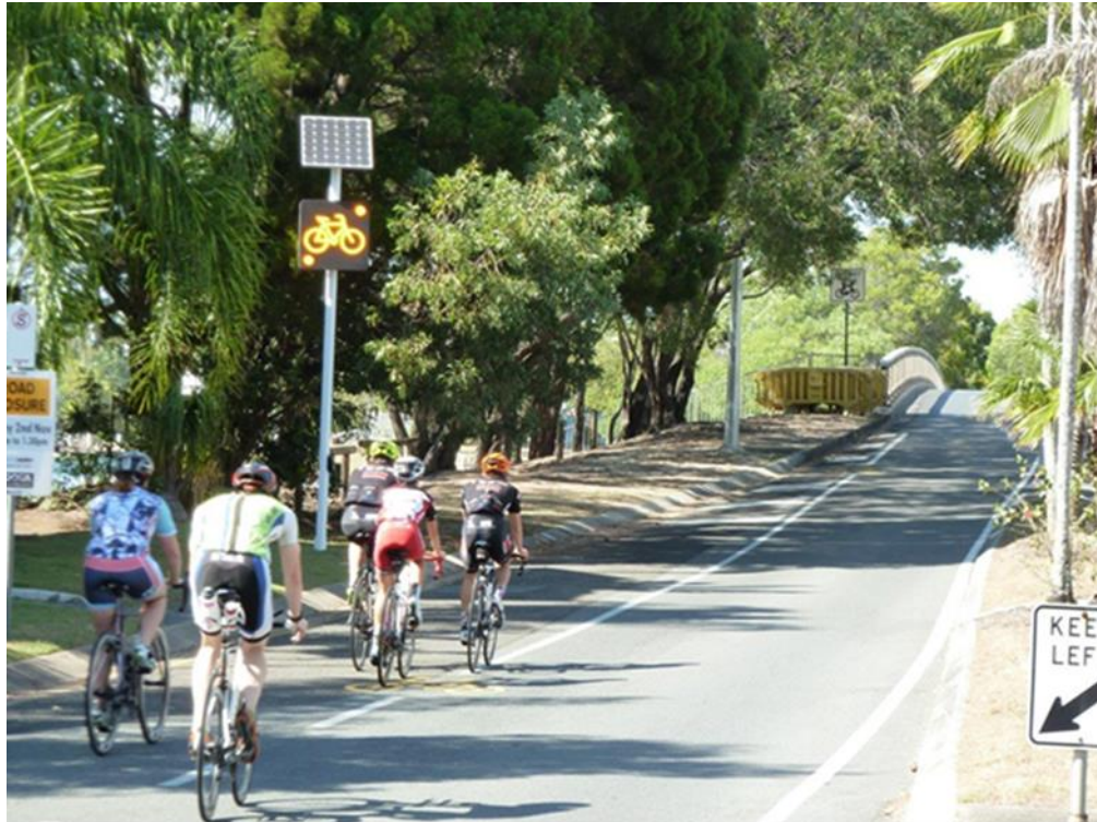
Figure 8(C) – Narrow bridge (no shoulder), Noosa Parade, Munna Point Bridge, Noosa Heads, Australia
