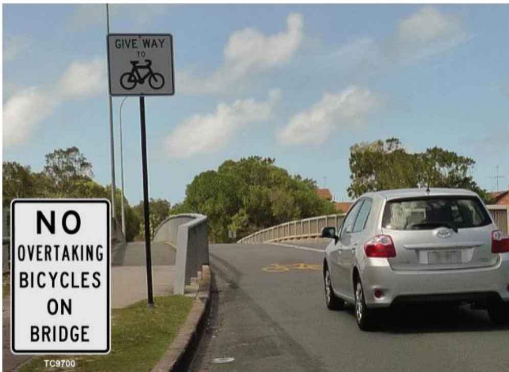
Figure 2.3(D) – Narrow bridge
