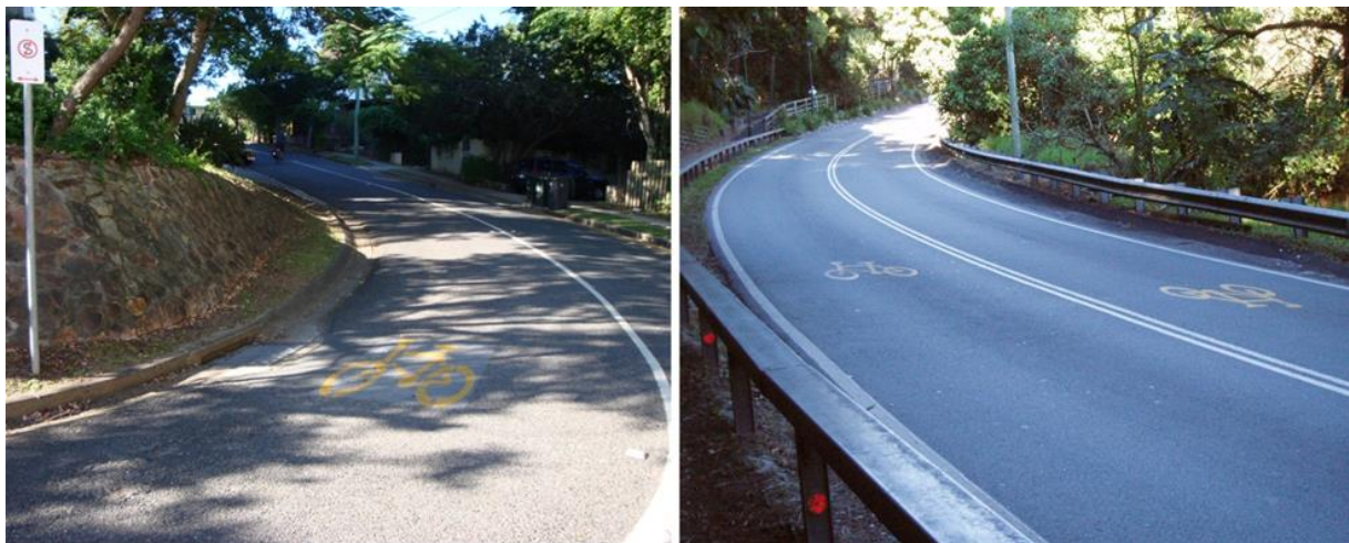
Figure 2.3(G) – Narrow road lanes on sight-restricted corners
