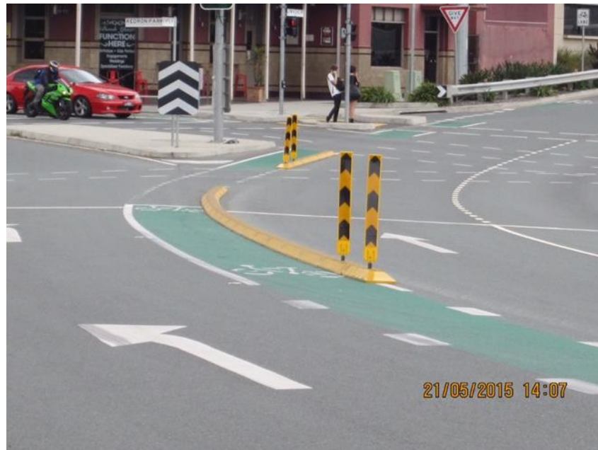
Figure 4.1.2(C) – Gympie Road at Kedron Park Road southbound, Kedron Park (plastic kerb with vertical delineators)
