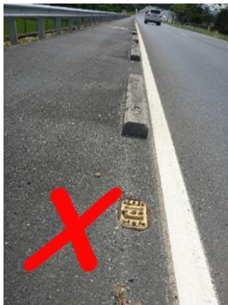
Figure 3 – Example of historical concrete barrier kerbs
