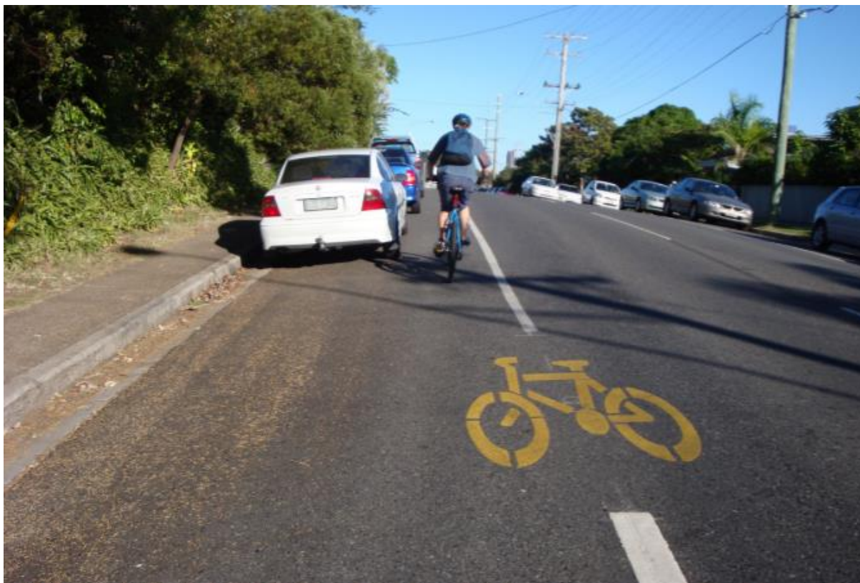
Figure 2.4(B) – Inappropriate application of a Bicycle Awareness Zone in the ‘door zone’
