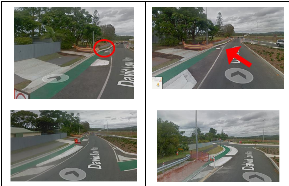
Figure 4.1.1 – David Low Way: Showing concrete islands separating the bicycle lane from the road
