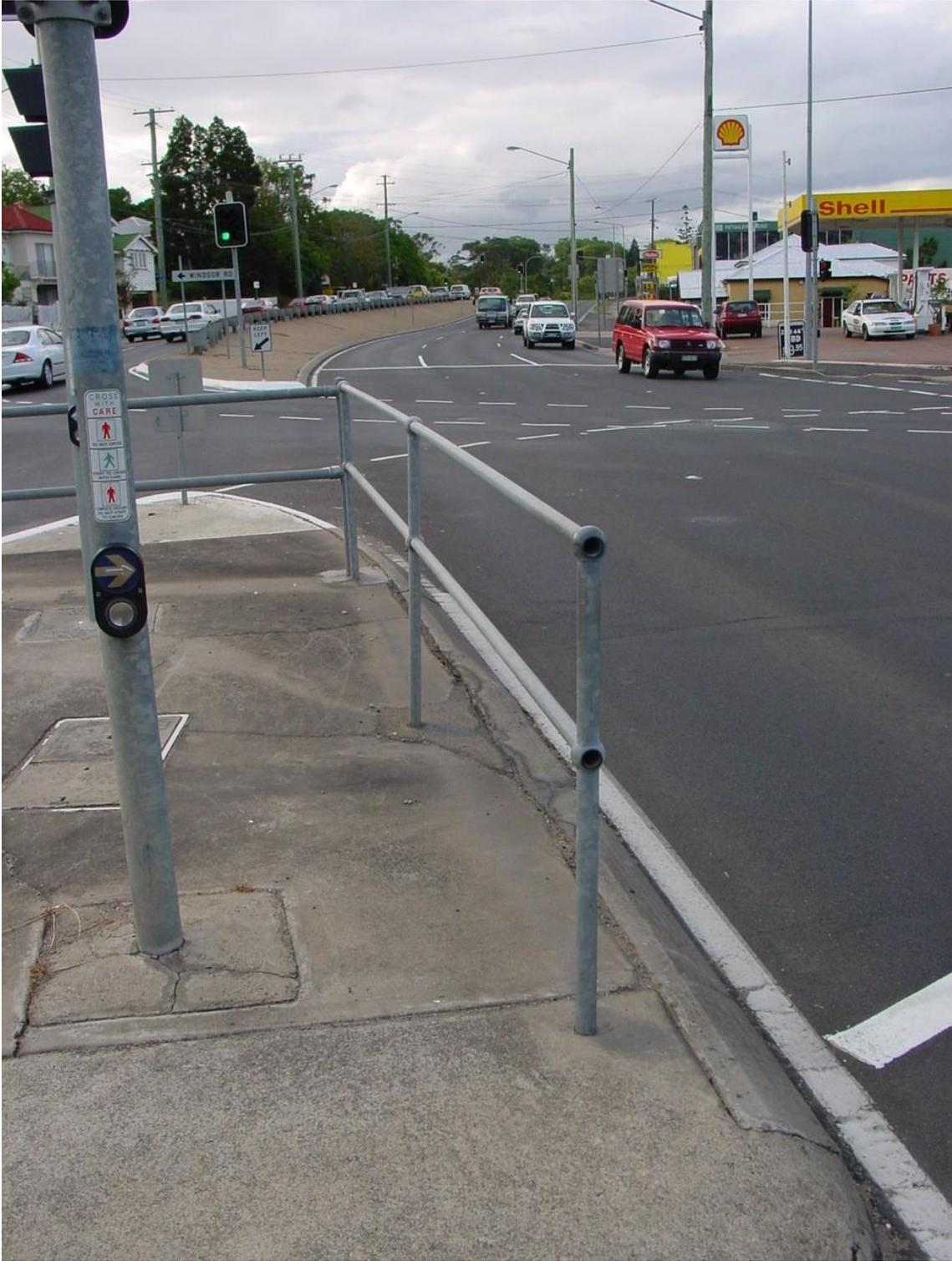
**Figure 1.1-E – Pedestrian fences, when installed at medians, should commence at the signal post and not encroach past the push button position**
