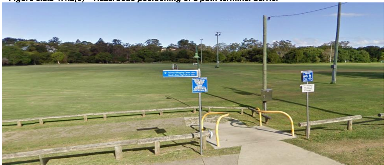
Figure 8.2.2-1.1.2(5) – Hazardous positioning of a path terminal barrier
