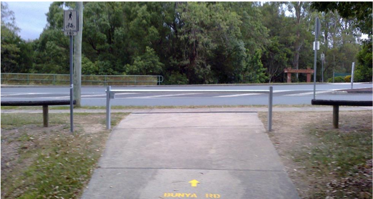
Figure 8.2.2-1.1.2(7) – Hazardous path terminal device, limited visibility due to lack of contrast
