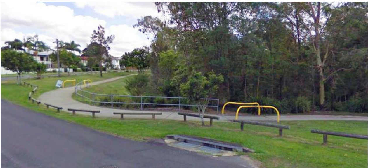
Figure 8.2.2-1.1.2(1) – Excessive use of physical barriers to slow cyclists on approach to a blind corner
