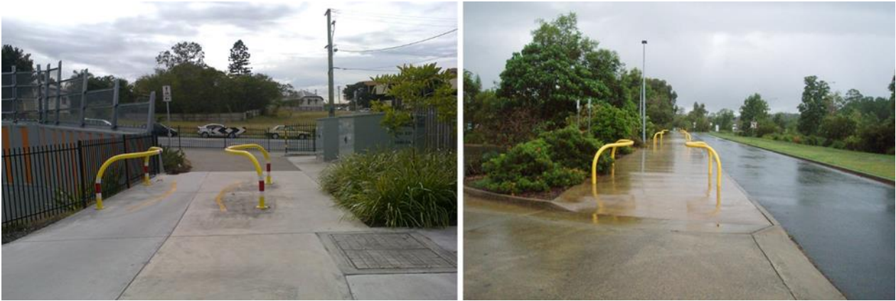
Figure 8.2.2-1.1.2(6) – Examples of easily avoidable and redundant physical barriers
