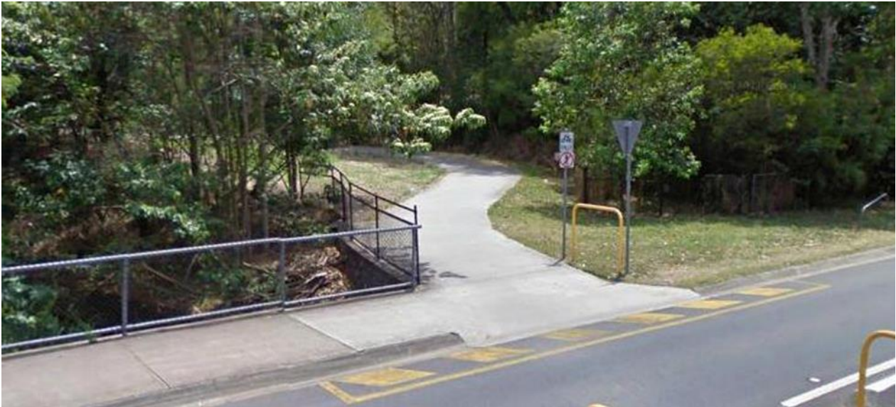
Figure 8.2.2-1.3.2(2) – Example of terminal appearance treatment using pavement markings
