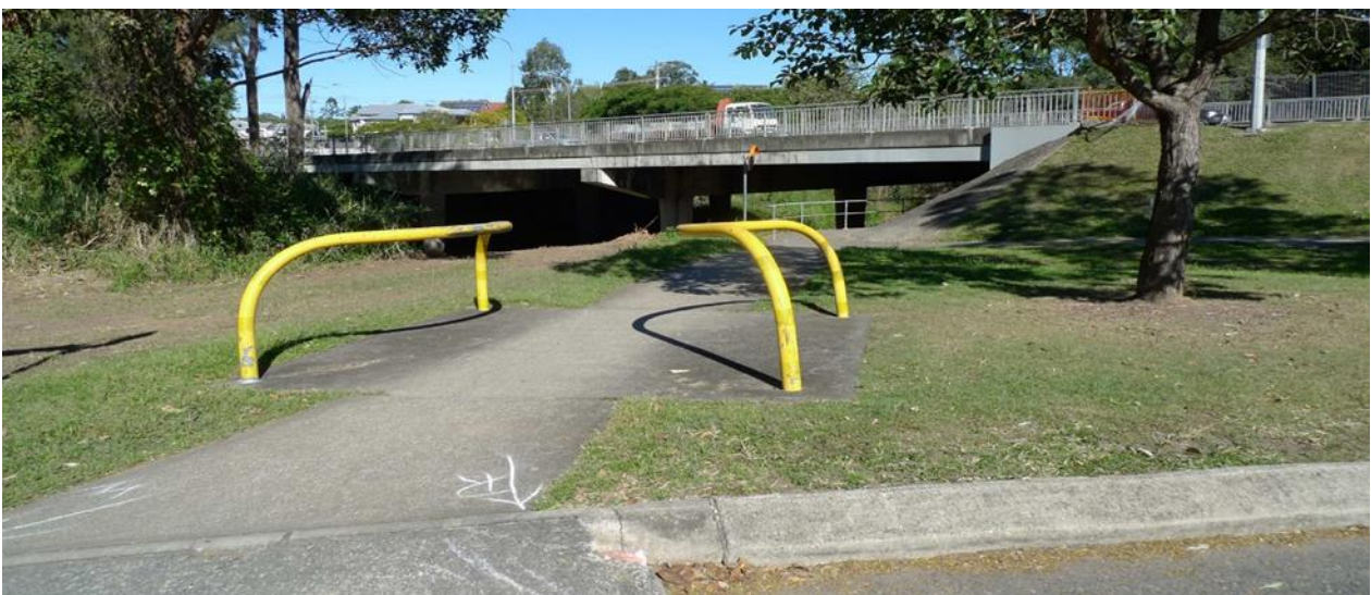
Figure 8.2.2-1.1.2(2) – Redundant path terminal barrier
