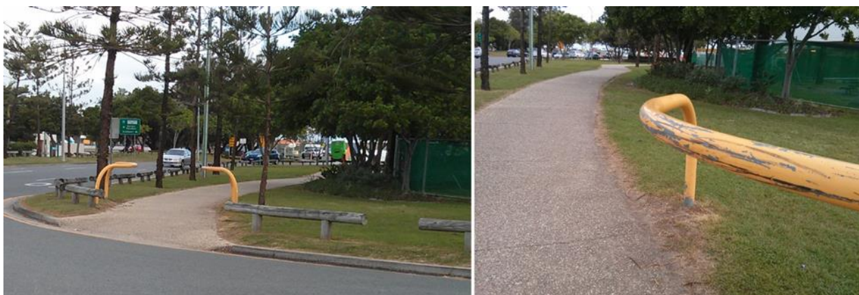
Figure 8.2.2-1.4.2(1) – Damage which indicates evidence of insufficient passing width
