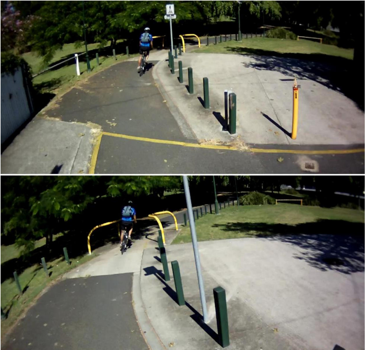
Figure 8.2.2-1.4.4 – Illustration of cyclists ‘lean into’ corner turns, and the hazardous positioning of this terminal barrier
