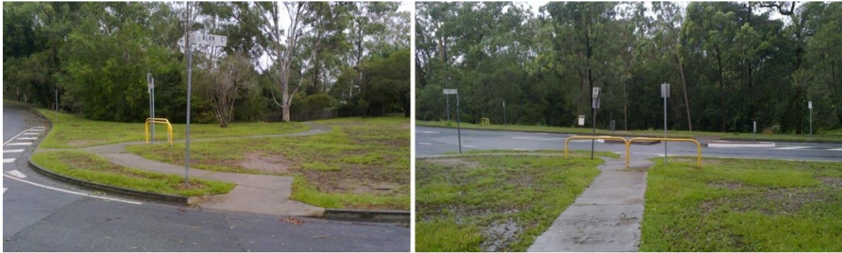
Figure 8.2.2-1.1.2(3) – Redundant U-rail type terminal barrier
