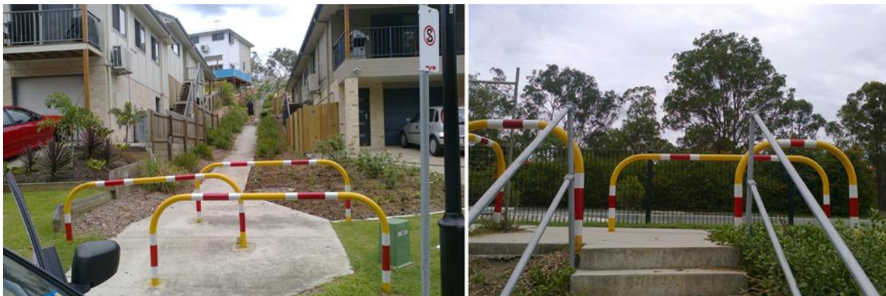
Figure 8.2.2-1.1.2(4) – Redundant U-rail type barrier on a set of stairs
