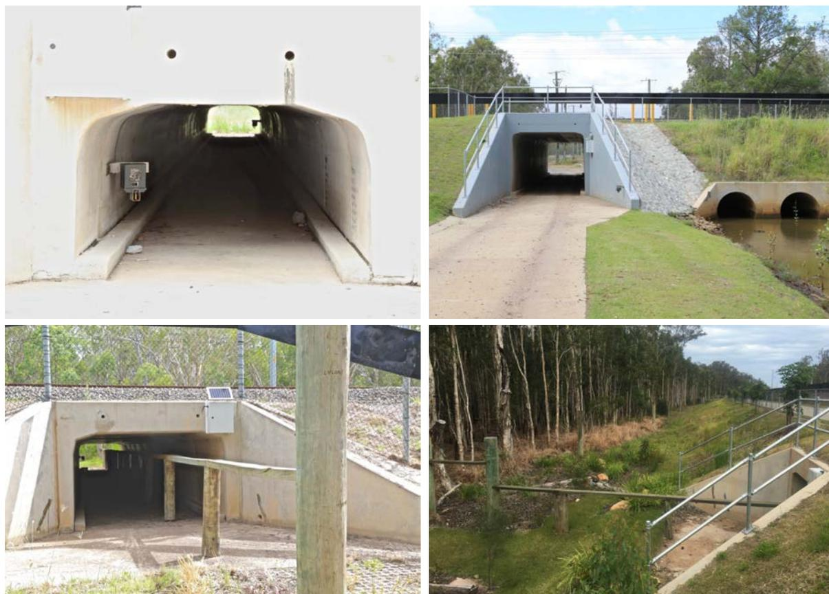
**Plate 3.14:** (Clockwise from top left) View through M31 (Kippa-Ring) showing outward-facing trail cameras installed at either end (Trail cameras are Reconyx® PC900 professional series cameras with heavy duty anti-theft security boxes and brackets.); V2 at Kippa-Ring with M28 wet culvert on the far right; view of the northern opening of F3 (Kippa-Ring) showing landscaping and fauna furniture; F5 southern opening, showing fauna furniture and data-logger.
