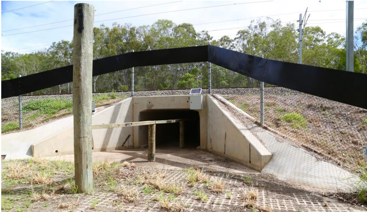
**Plate 6.3.** Five dedicated fauna culverts were installed beneath the rail corridor to provide corridor permeability and retention of some ecological connectivity between koala habitat. Post-and-rail fauna furniture provided opportunities for safe passage / travel off the ground for koalas, although they were more commonly used by possums.
