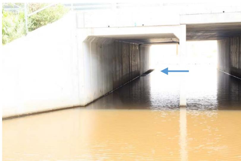
**Plate 12.14:** Photo of the eastern opening of the southern box culvert under Brays Road. The fauna ledge is visible at the rear of the culvert (arrow), but dives down under the water level, such that it is submerged by approximately 400mm at its eastern termination. Hence, its functionality as a dry-passage fauna ledge is completely obviated.
