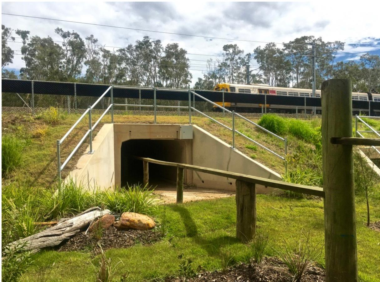
**Plate 3.12:** Fauna culvert F3 at Kippa-Ring with fauna furniture and entry landscaping. Fauna fencing can be seen in the background with the black anti-climb sheeting. Drainage culvert M29 is just visible in the far right of the photograph. Both culverts were used by koalas and a variety of other fauna to transit the rail corridor.
