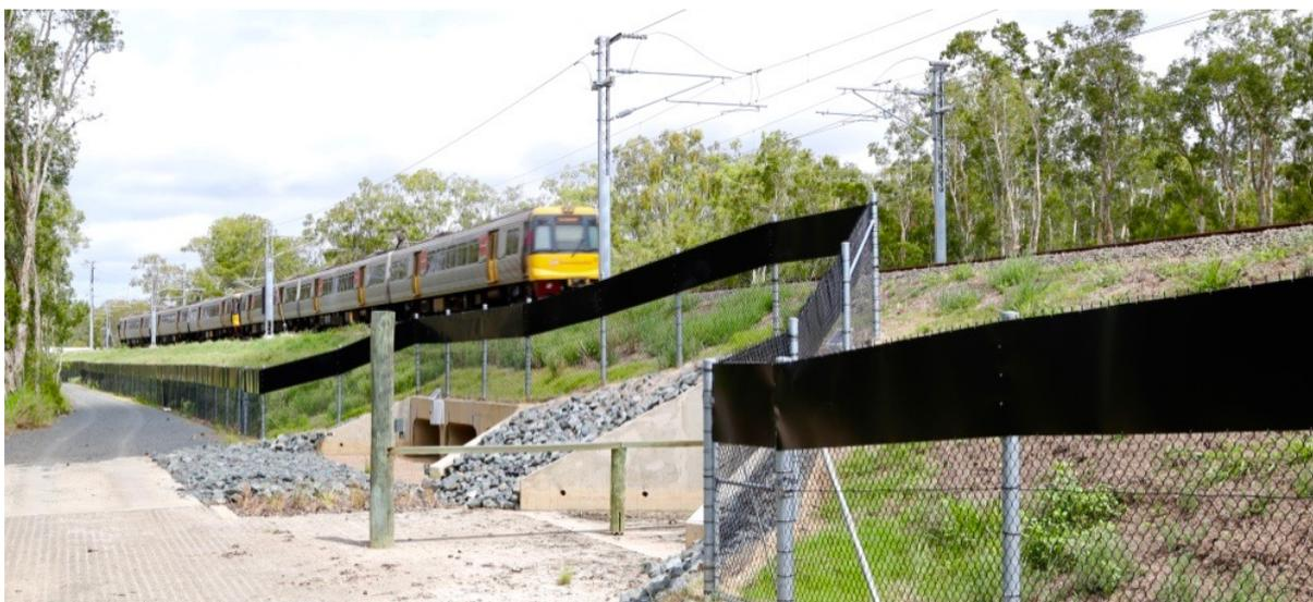
**Plate 3.4:** The proper design, installation and maintenance of fauna exclusion fencing and effective barrier-crossing structures, can very significantly reduce mortality and other adverse ecological impacts of linear infrastructure. This image shows properly installed mammal exclusion fencing, and two effective crossing structures - a drainage culvert (M29) and a dedicated fauna culvert (F3) in a section of the Redcliffe Peninsula Line transecting wildlife habitat at Kippa-Ring.
