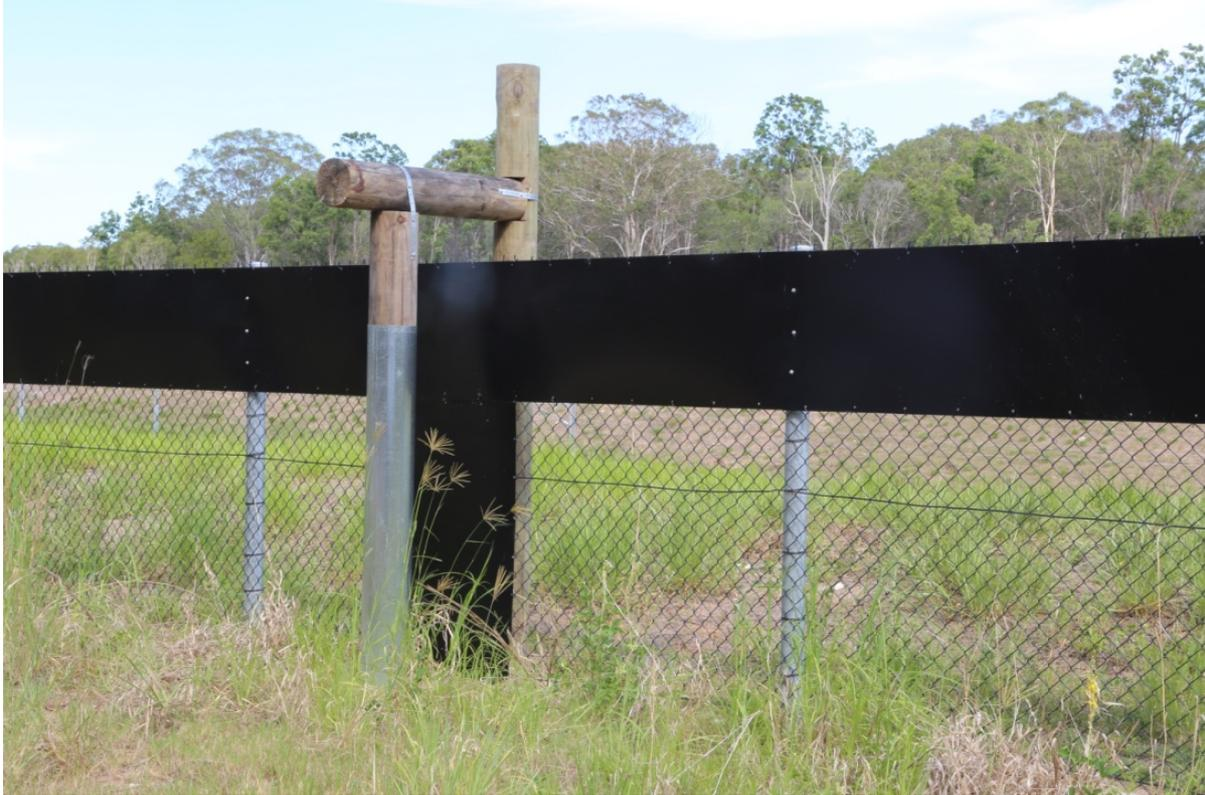
**Plate 3.15:** Fauna exclusion fencing along the rail corridor at the Amcor site, with escape-pole egress device. Egress poles are probably less effective for koalas than ground-installed egress valves (see below) due to the cognitive processes of a koala traversing the ground.
