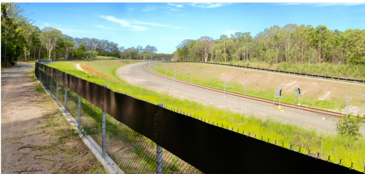
**Plate 3.16:** Fauna fencing along the rail boundary at the large cut through the Amcor site. This section has limited crossing opportunities for wildlife, with an approximately 1km span between crossing structures at Yebri Ck and the drainage culvert M12 near Dohle's Rocks Road. The barrier-effect of this section of the rail line remains relatively unmitigated.
