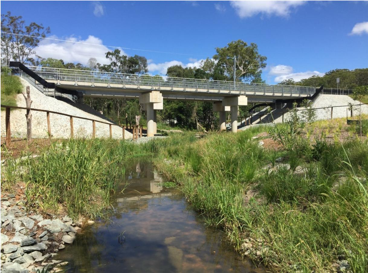
**Plate 6.4:** Bridges such as the new Yebri Creek Rail bridge on the Amcor site provides suitable safe passage under the rail line for koalas and other fauna where dry areas exist. Elevated passage using post-and-rail structures is available on both sides of the creek. These were commonly used by brushtail possums.
