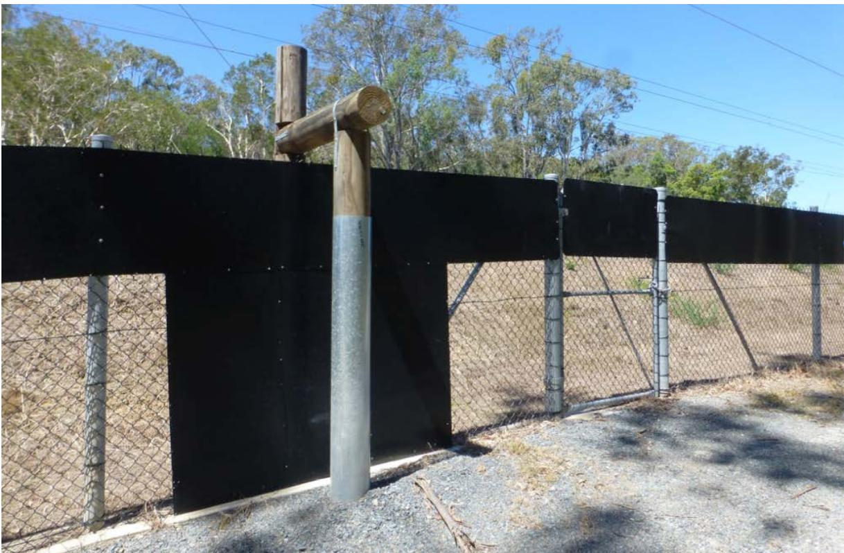
**Plate 6.5:** Koala proof fencing consists of chain wire fencing with a 600mm wide sheet of non-climbable sheet-metal attached to the top of the fence. The fencing serves the dual purpose of funnelling koalas to dedicated safe fauna crossing structures beneath the rail corridor and mitigating the risk of koala mortality from train strike. This photo also shows an escape pole designed to facilitate the exit of a koala from the rail corridor.
