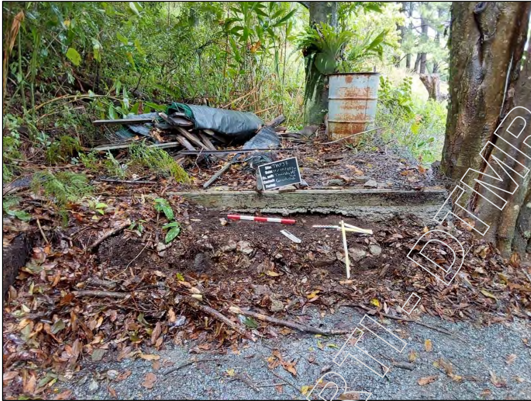
Figure 7 – northern end of the concrete slab showing the underlying soil profile and macadamia tree
