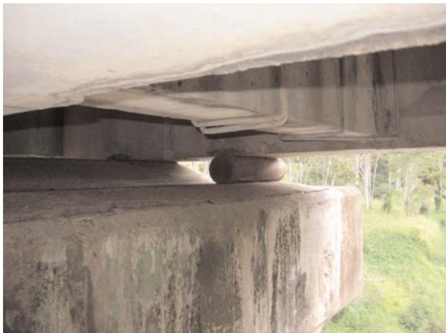
**Photo 3: Steel Roller bearings and poor drainage provision on headstock**
