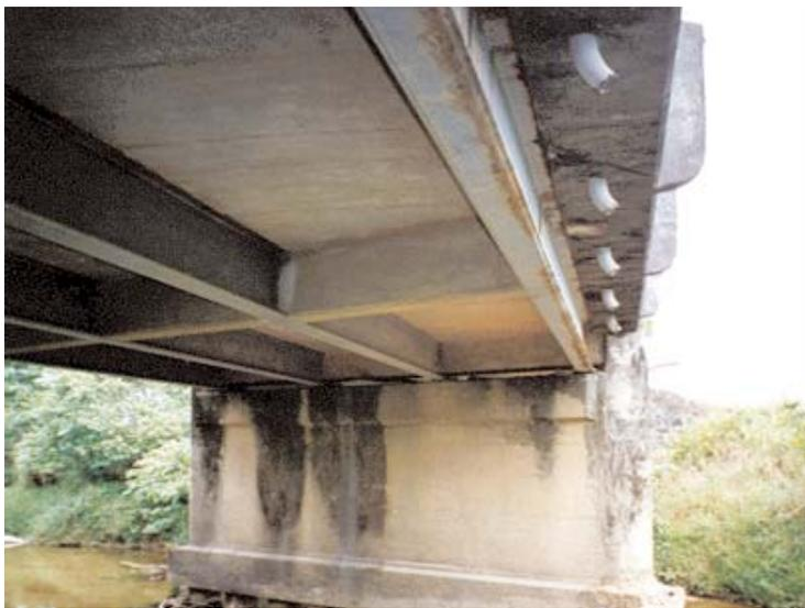
**Photo 6: Poor drainage detailing leading to corrosion of outer girder and staining on pier.**
