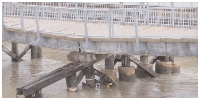
**Photo 1: Structural Failure due to degradation of timber piers**
