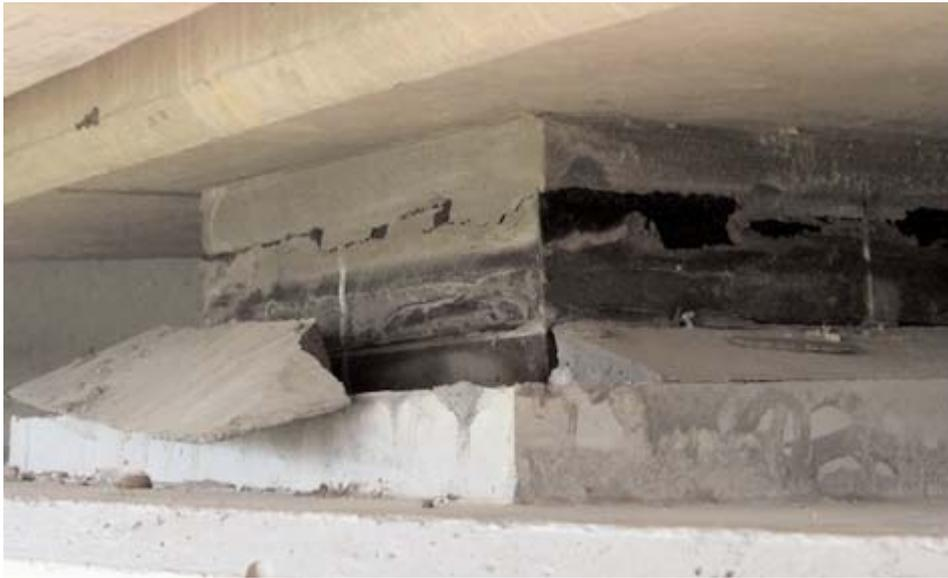
**Photo 7: Inadequate fixity around elastomeric bearing**
