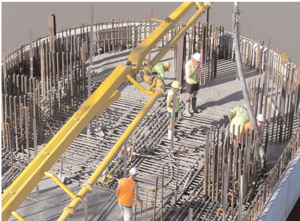
*Photo 8: Concrete placement in a pier*
