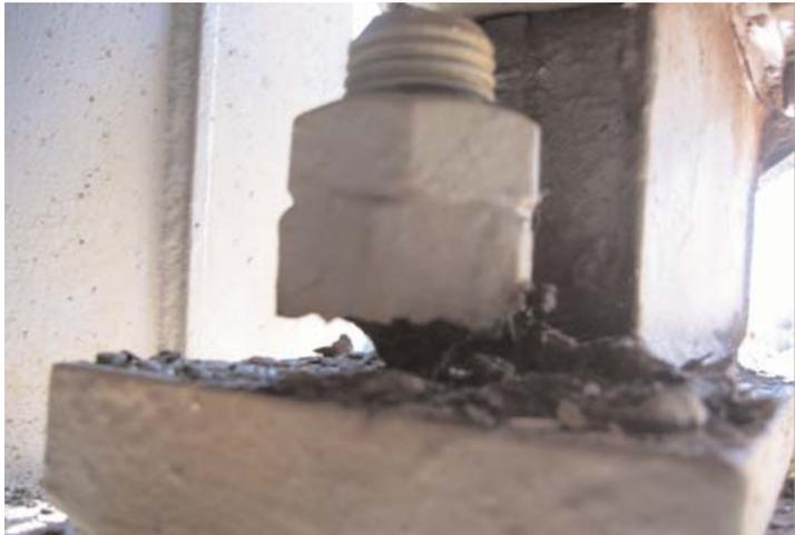
**Photo 5: Corrosion resulting in necking of holding down bolt**
