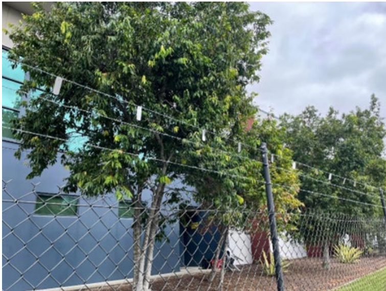
Figure 7.1 – Reflective disks on barbed wire fencing may increase the visibility of the fence to flying-foxes and reduce entanglements
