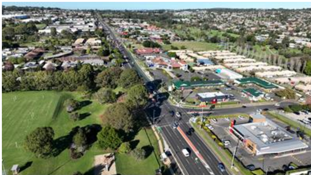
New England Highway, Ruthven Street, Toowoomba
