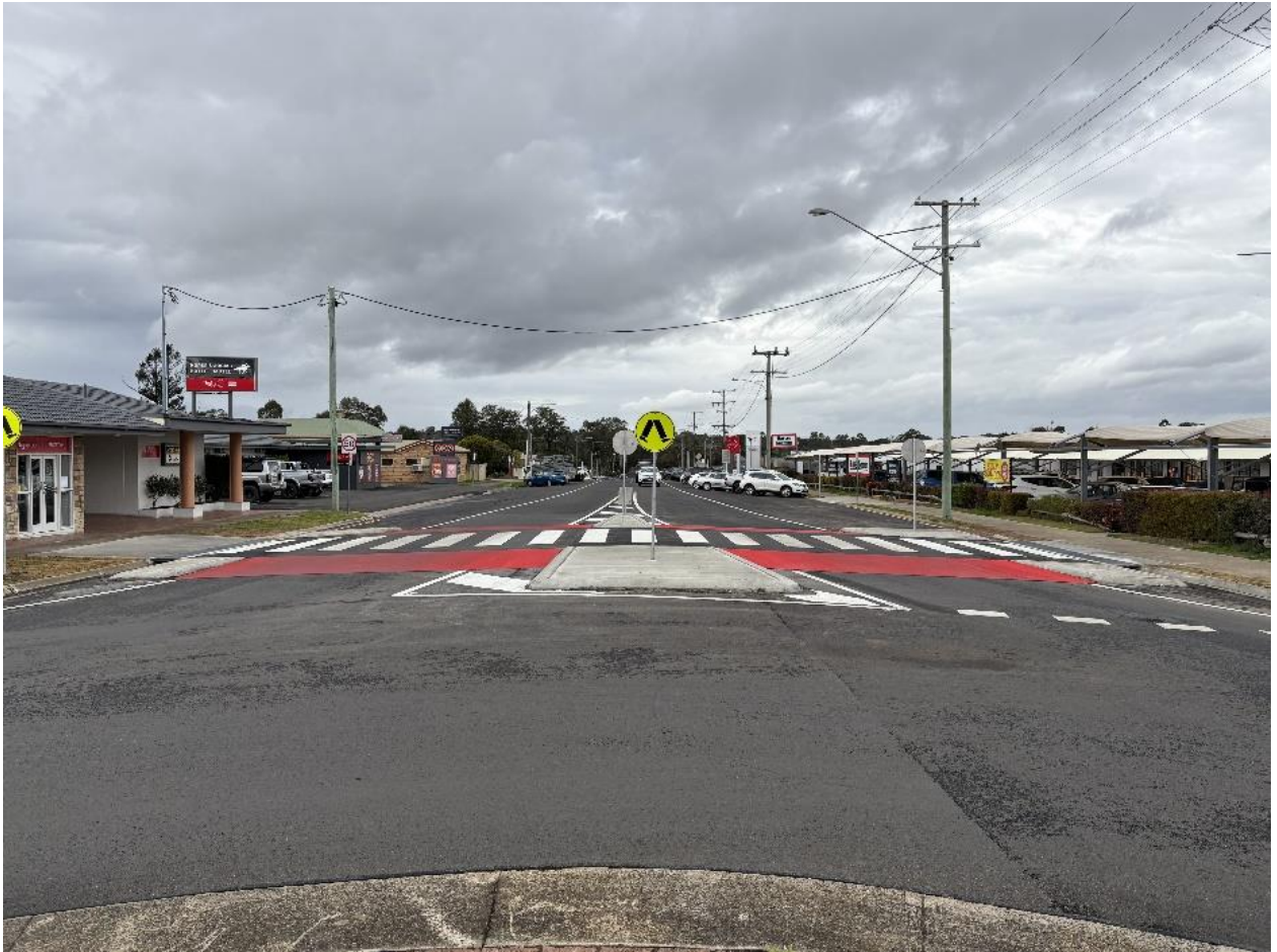
Wombat crossing installed on Victoria Street
