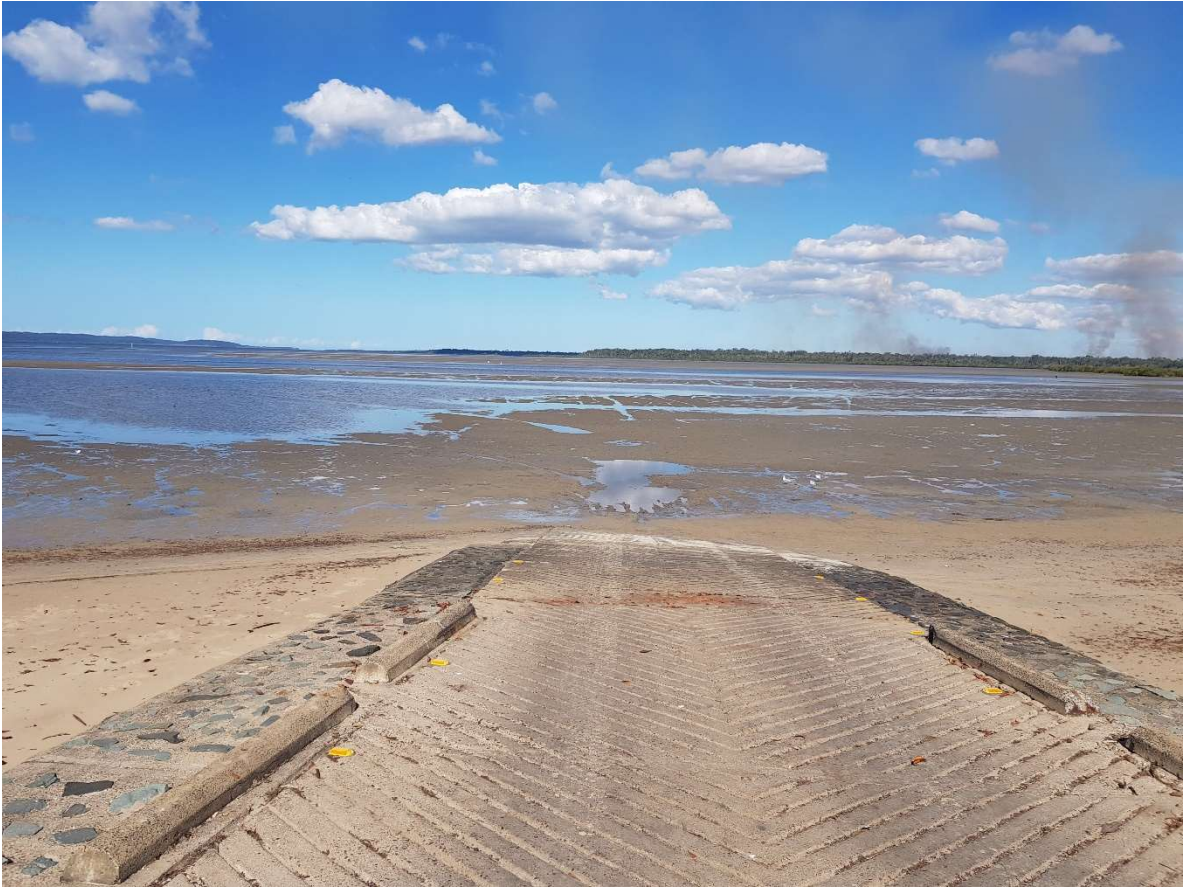
Image 1 – Poona Boat Ramp existing boat ramp facility
