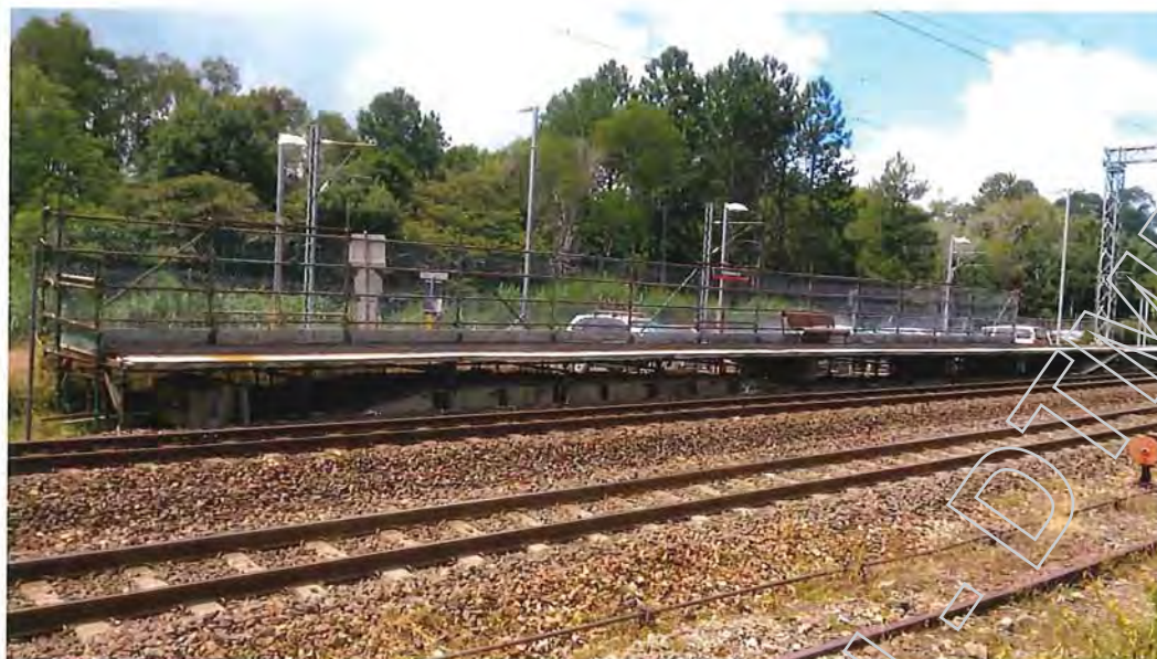
Above: Palmwoods Station Platform with temporary platform extension on scaffolding
