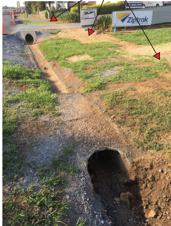
Line of council water main excavation
