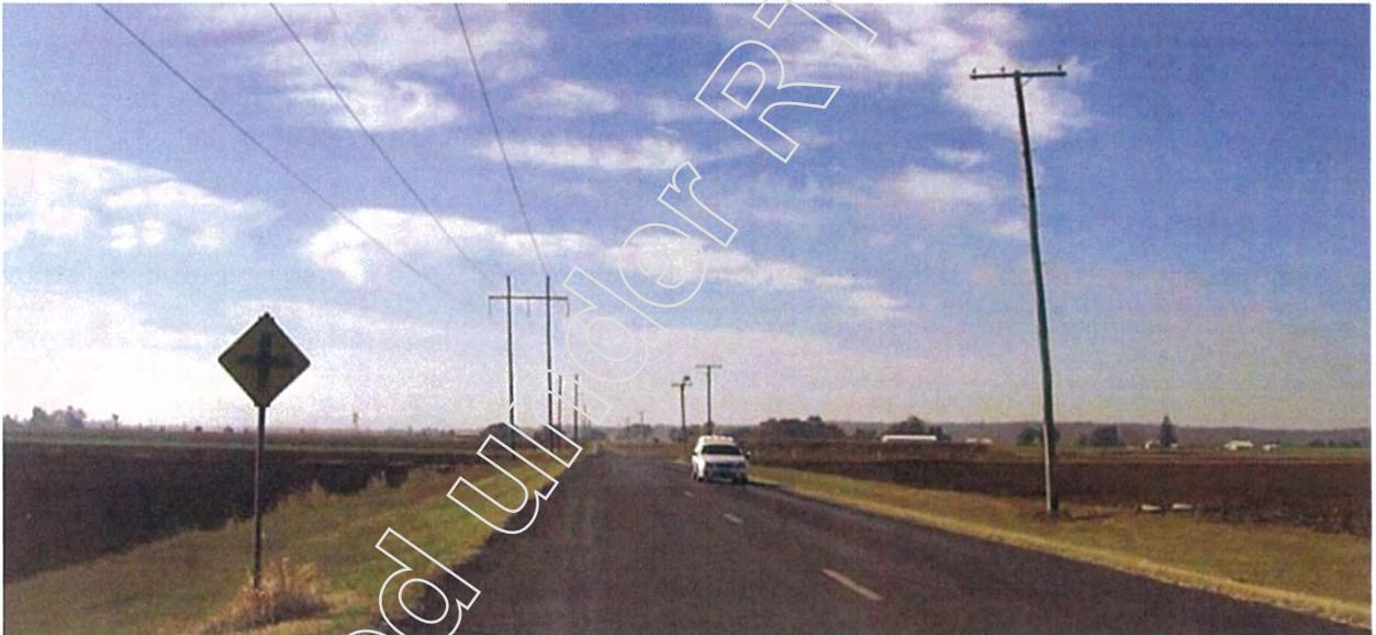
Figure 12 – Lake Clarendon Way – Westbound Approach – Faded Advance Intersection Warning Sign
