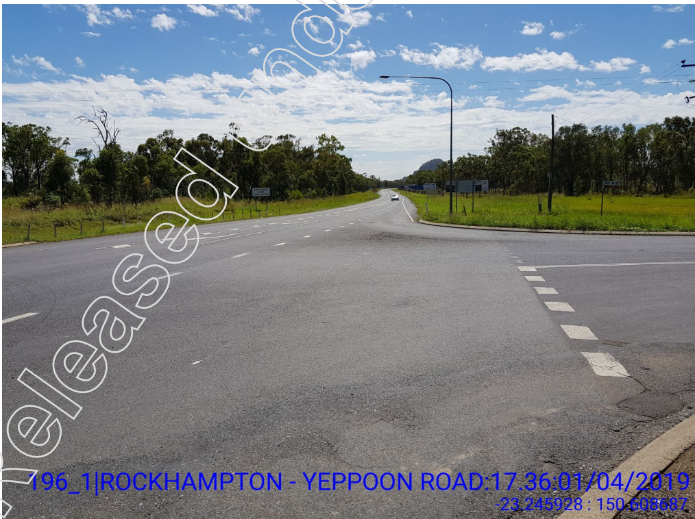
Looking north-east from the southern corner of Dairy Inn Road and Rockhampton-Yeppoon Road, note fatigue cracking and patching in the pavement in the left-out turning area of the intersection
