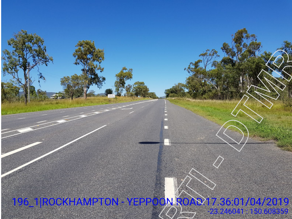
Looking back down the road towards the south-west, at the turnoff onto Artillery Road. Note linemarking is in good condition
