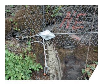
TECCO®-Slope Stabilization (Anchorage of Border Rope)
