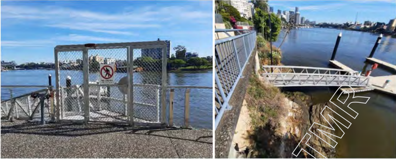
Figure 18: Access to existing pontoons via locked gate (Mon Reve, left) and underpass (Dundrenan Residences, right)
