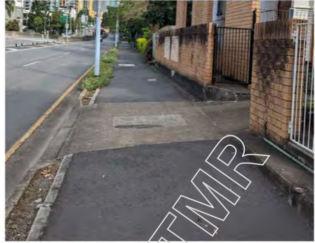
Figure 4: Existing verge crossfall – Shafston Ave
