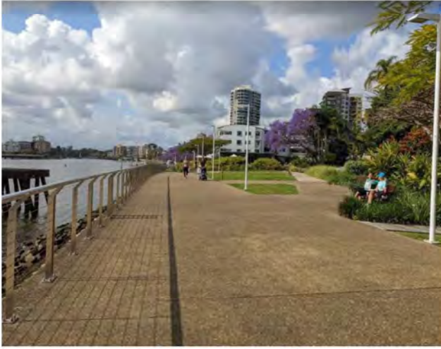
Figure 6: Riverside with steel balustrade
