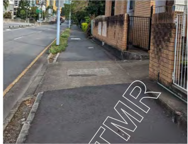
Figure 4: Existing verge crossfall – Shafston Ave
