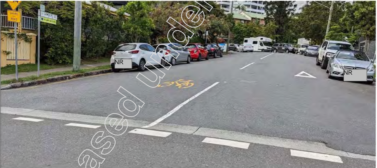
Lambert Street / Cairns Street intersection: Spoon drain.
