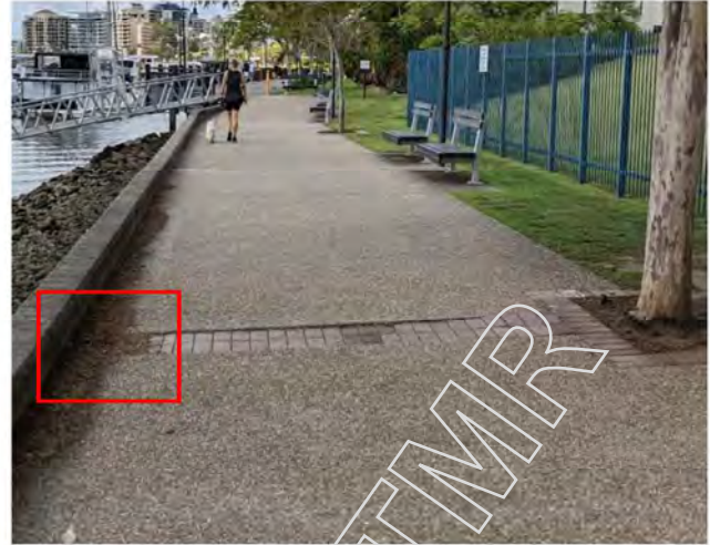
Figure 7: Riverside with concrete wall and blocked inlet
