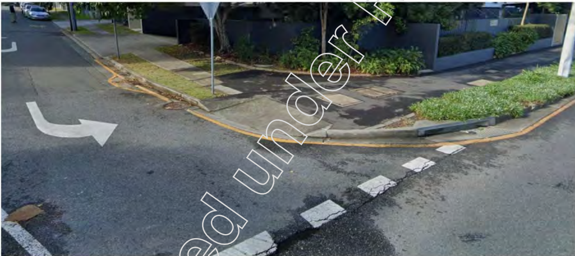
Figure 5: Kerb ramp with gully pit
