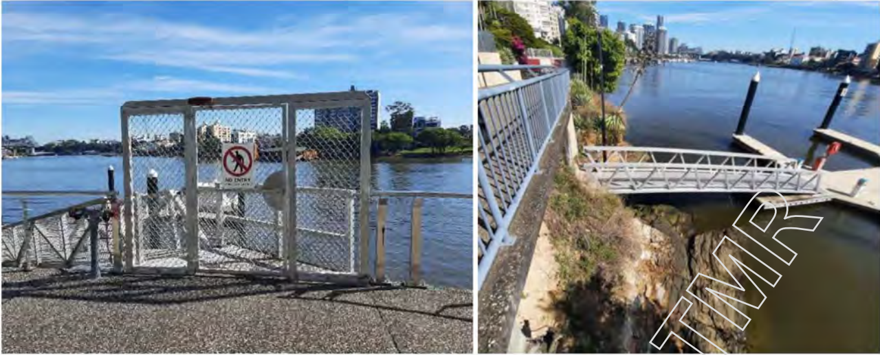
Figure 17: Access to existing pontoons via locked gate (left) and underpass (right)
