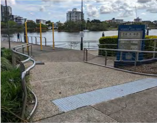
Figure 3: Ramp to promenade – Mowbray Park Ferry
