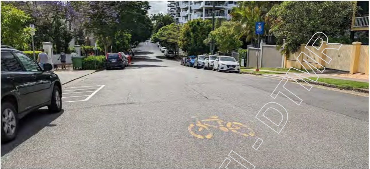
Cairns Street: View of the vertical grades present along Cairns St.
