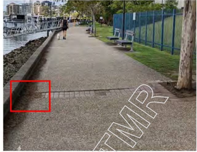
Figure 7: Riverside with concrete wall and blocked inlet
