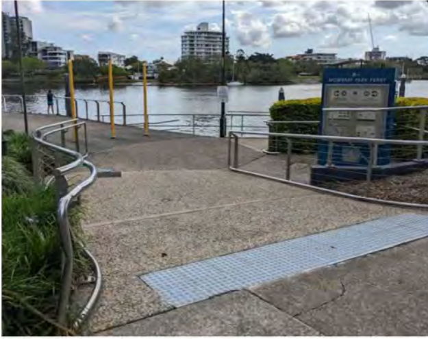
Figure 3: Ramp to promenade – Mowbray Park Ferry
