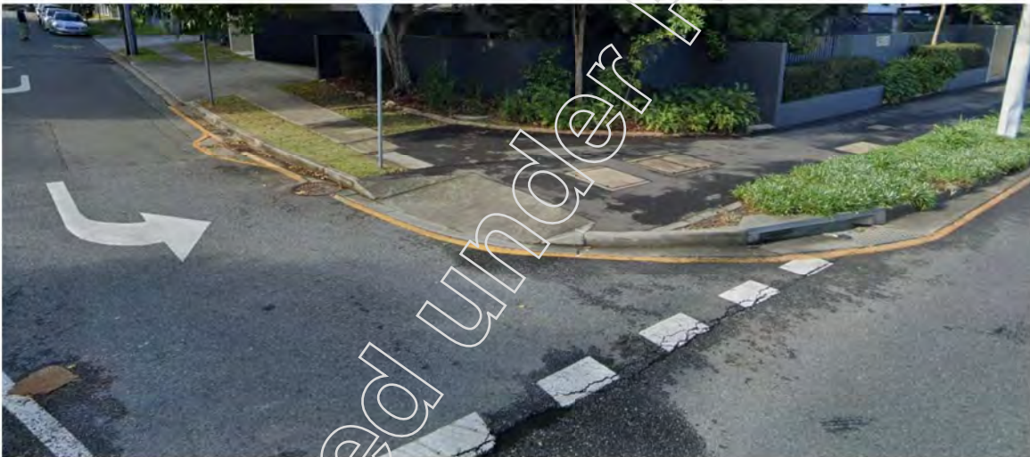
Figure 5: Kerb ramp with gully pit
