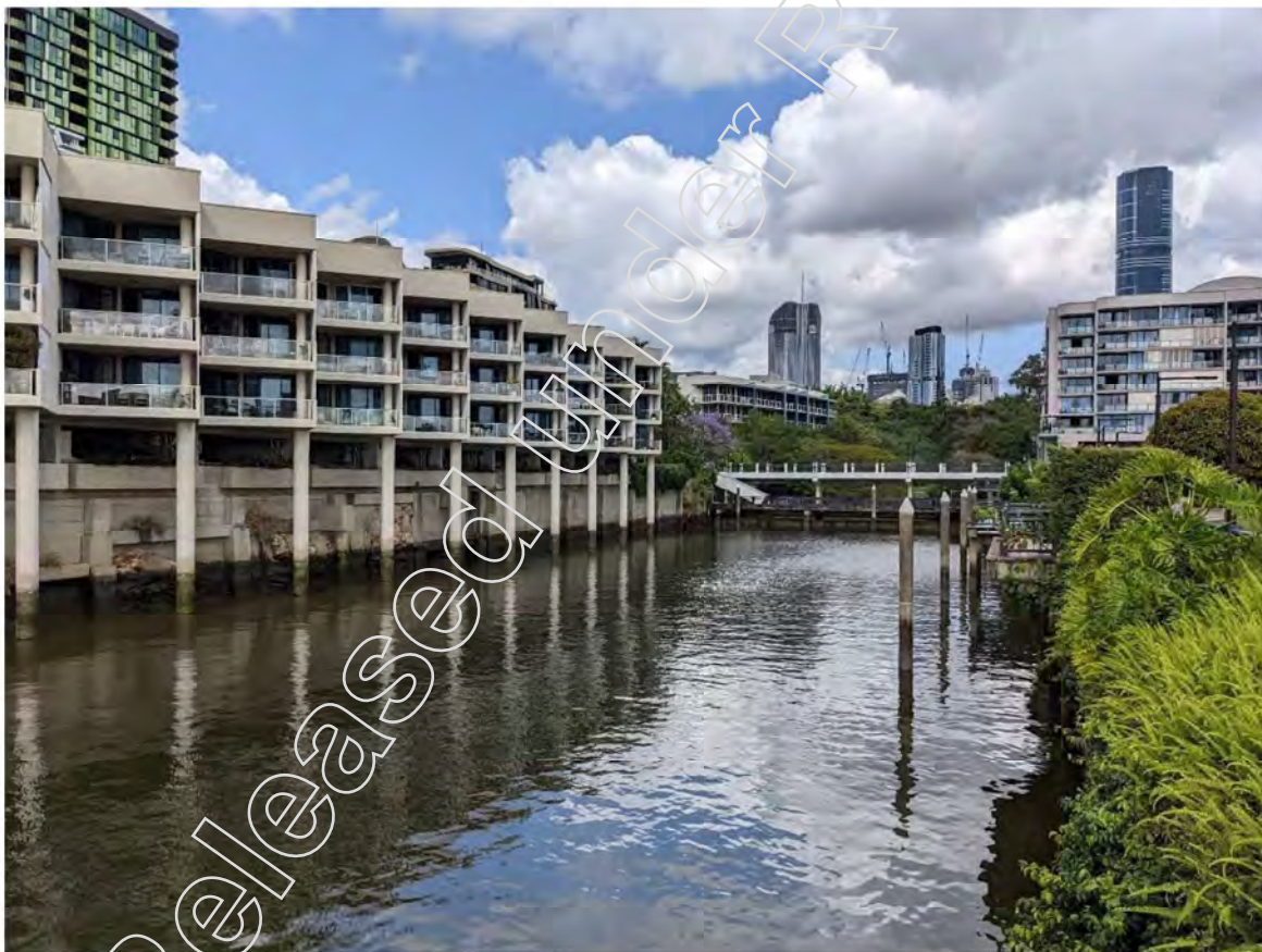
Figure 19: Existing condition of the former Dry Dock
