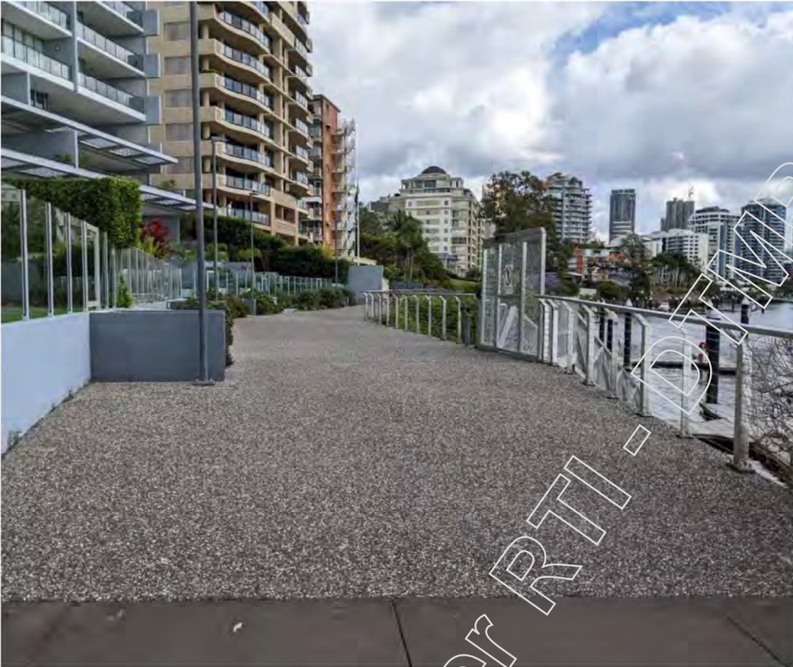
Typical promenade treatment exposed aggregate, stainless steel balustrade and raised adjacent blocks with retaining walls present.
