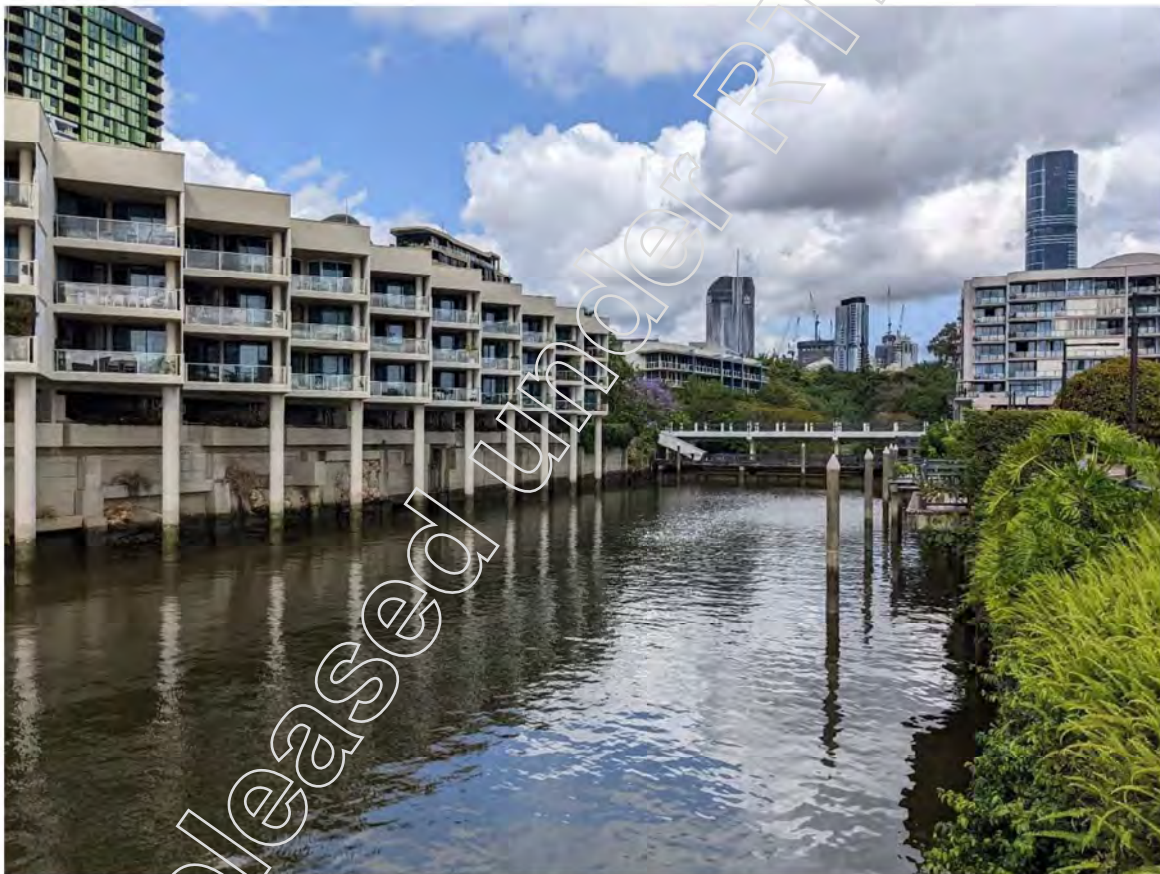
Figure 20: Existing condition of the former Dry Dock
