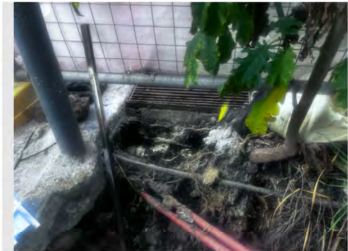
Description storm line out of pit in car yard
