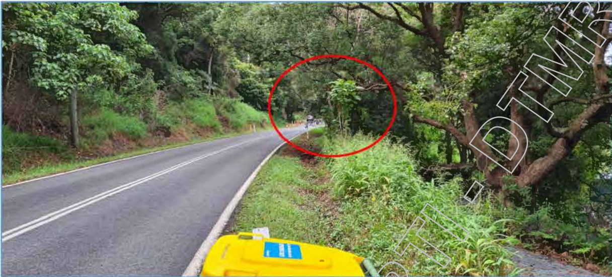
Figure 7: Vegetation Clearance at 628 Tomewin Mountain Road
