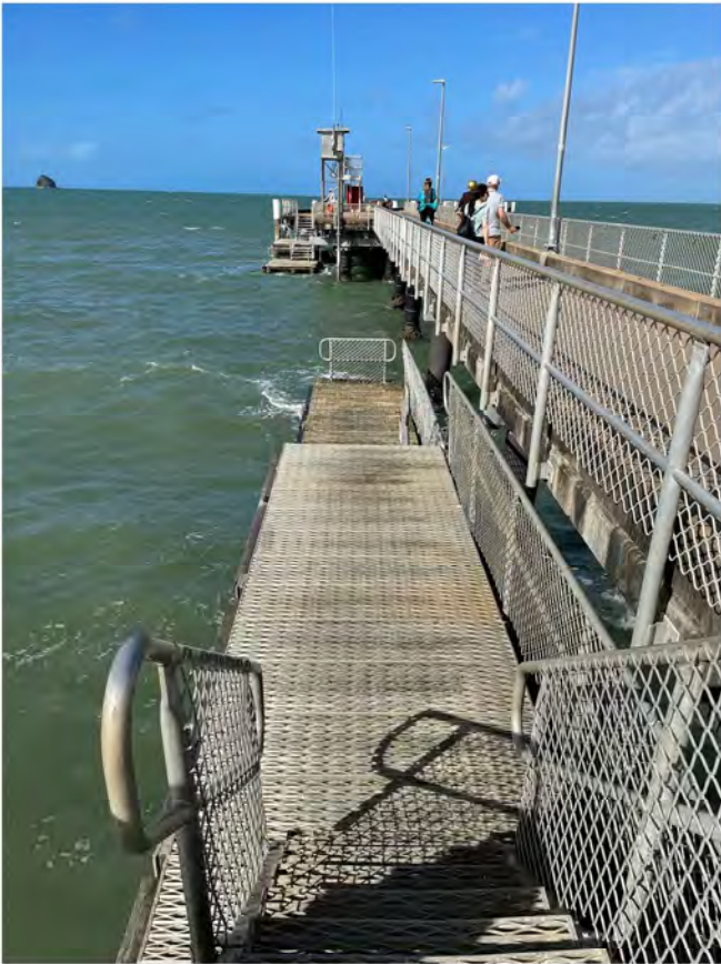
Figure 3 – Berth 2 stepped aluminium berth with lower landing removed and strip fendering
