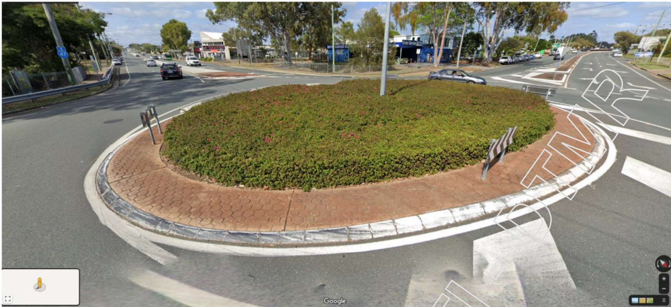
Figure 3.1 Existing centre island
