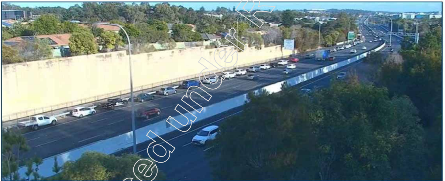
Figure 34 Exit 14: queues extend back to the motorway during morning peak period (07/08/24 at 7:45AM)
