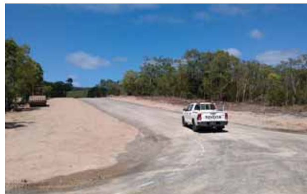
Pavement construction, Garden Street
