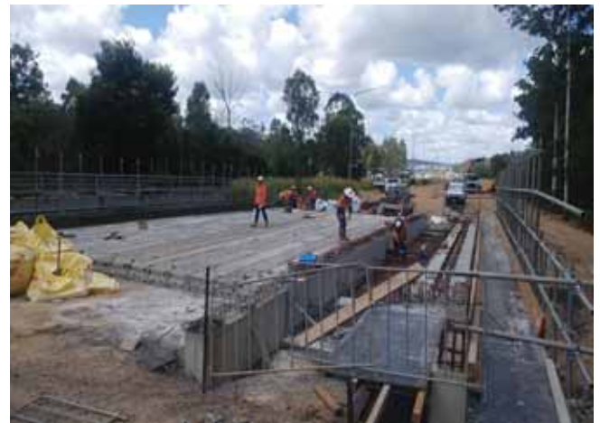
Springfield Greenbank Arterial Road and Springfield Parkway - bridge
