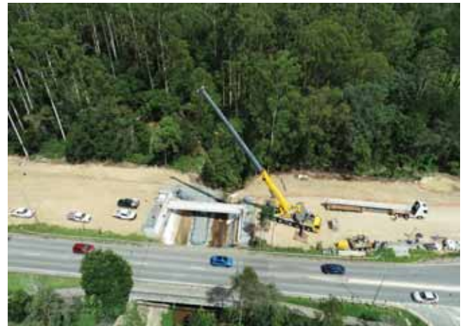
Springfield Greenbank Arterial Road and Springfield Parkway - bridge beams
