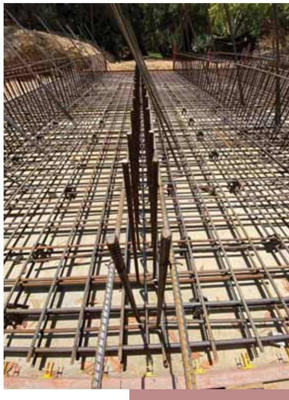
Magnificent Creek Overflow - reinforcement
