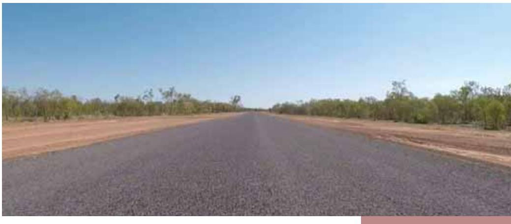
Richmond-Croydon Road - after (Ch 138)
