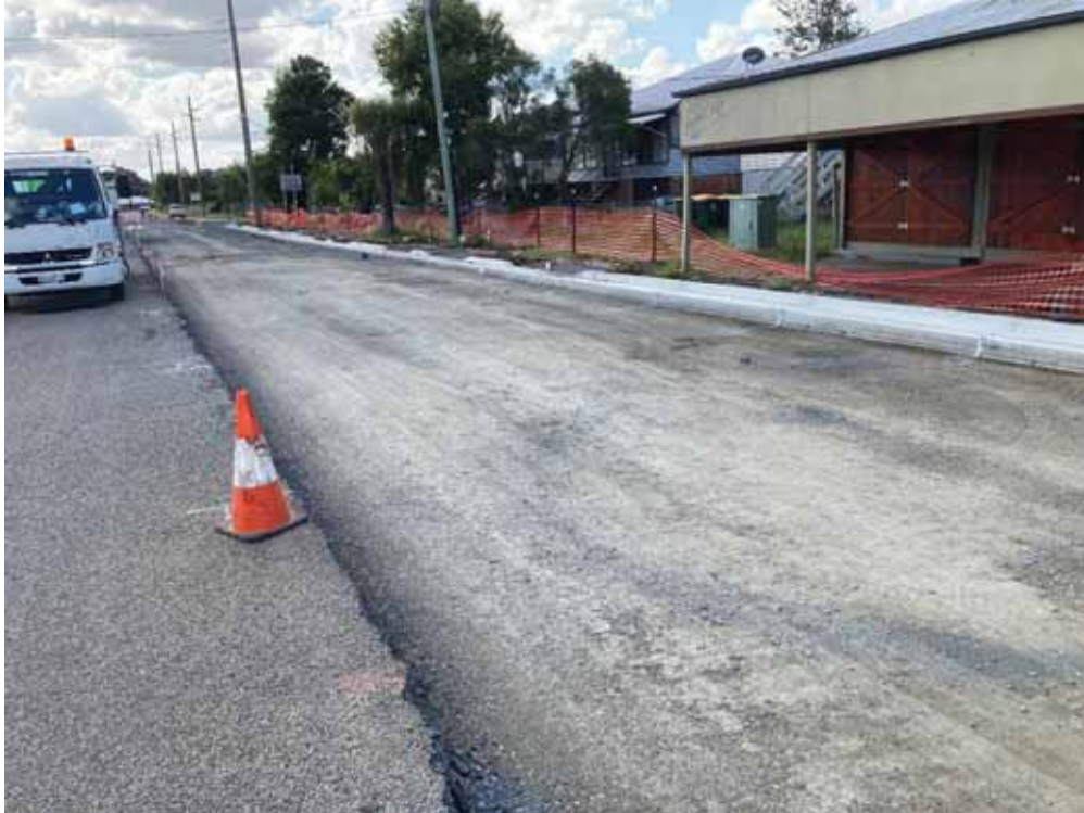
Glenmore Road - compacted subbase layer and new kerb and channel
