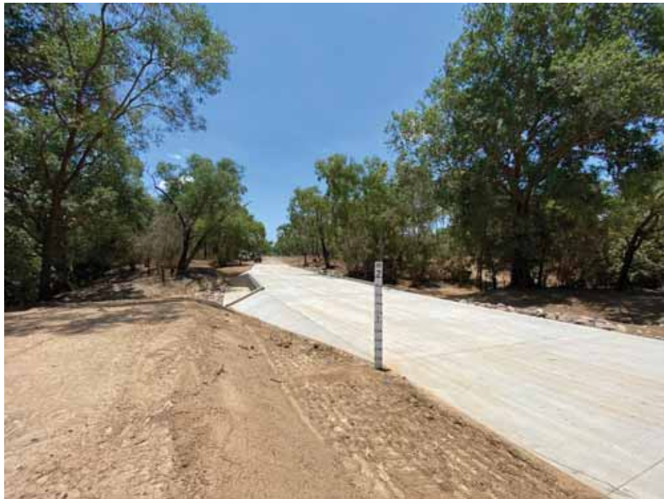
Magnificent Creek Overflow - completed
