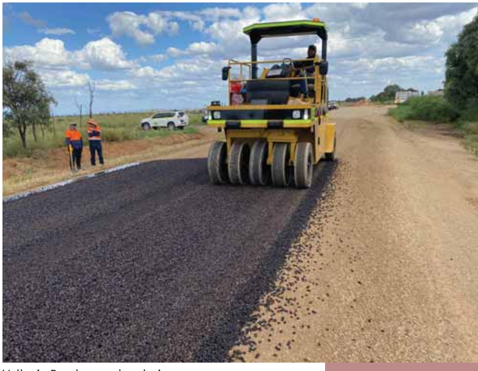
Valkyrie Road upgrade - during
