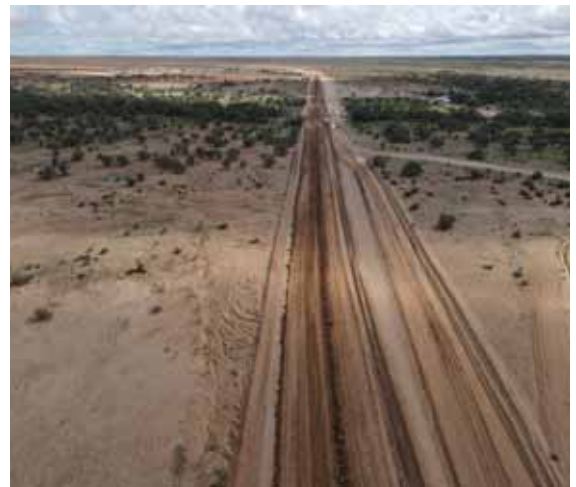
Bedourie-Birdsville - works underway
