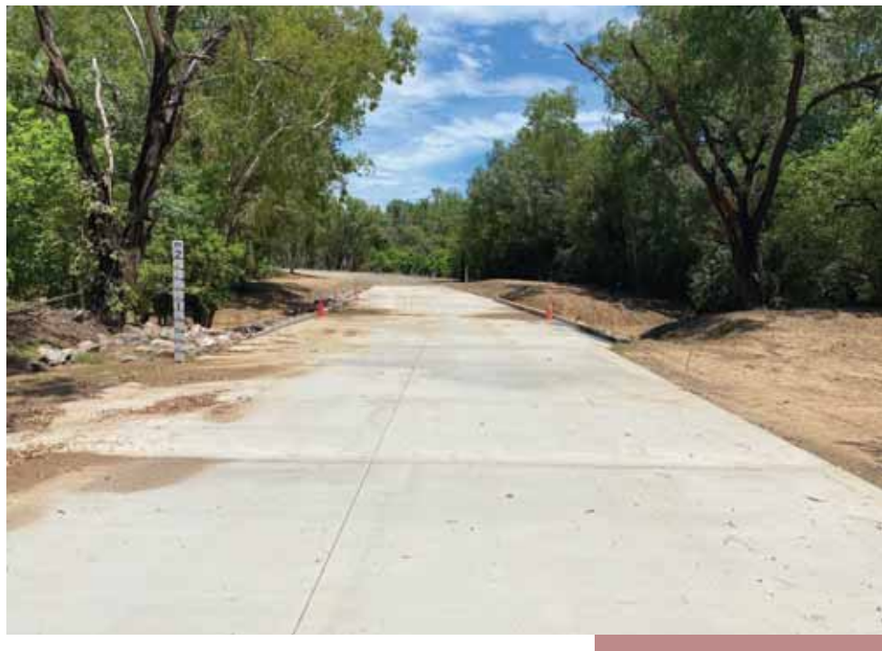
Magnificent Creek Overflow - taken after 2022 floods
