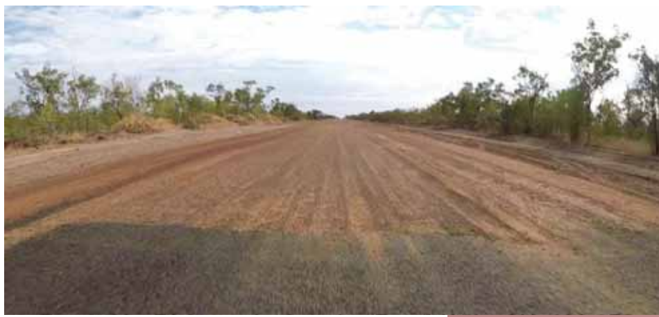
Richmond-Croydon Road - Before (Ch 126)
