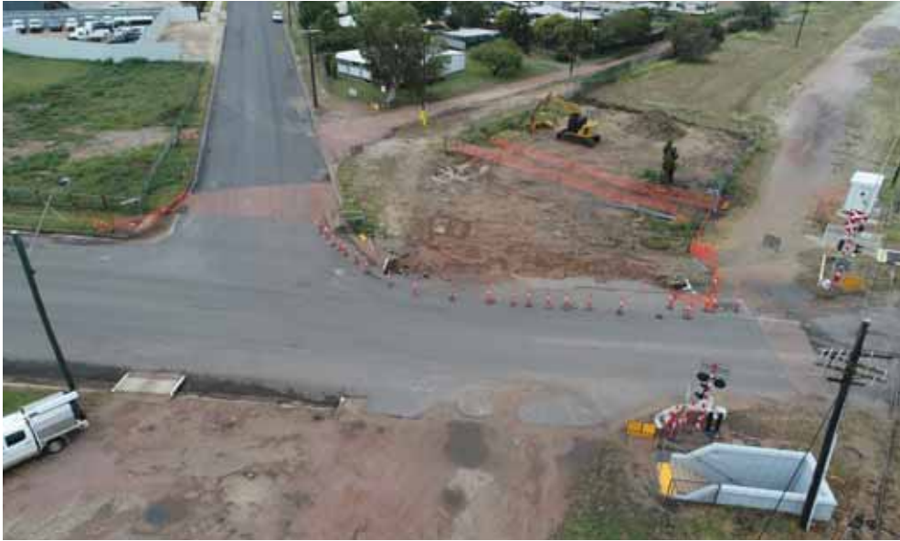
Victory Street-Millchester Road - during
