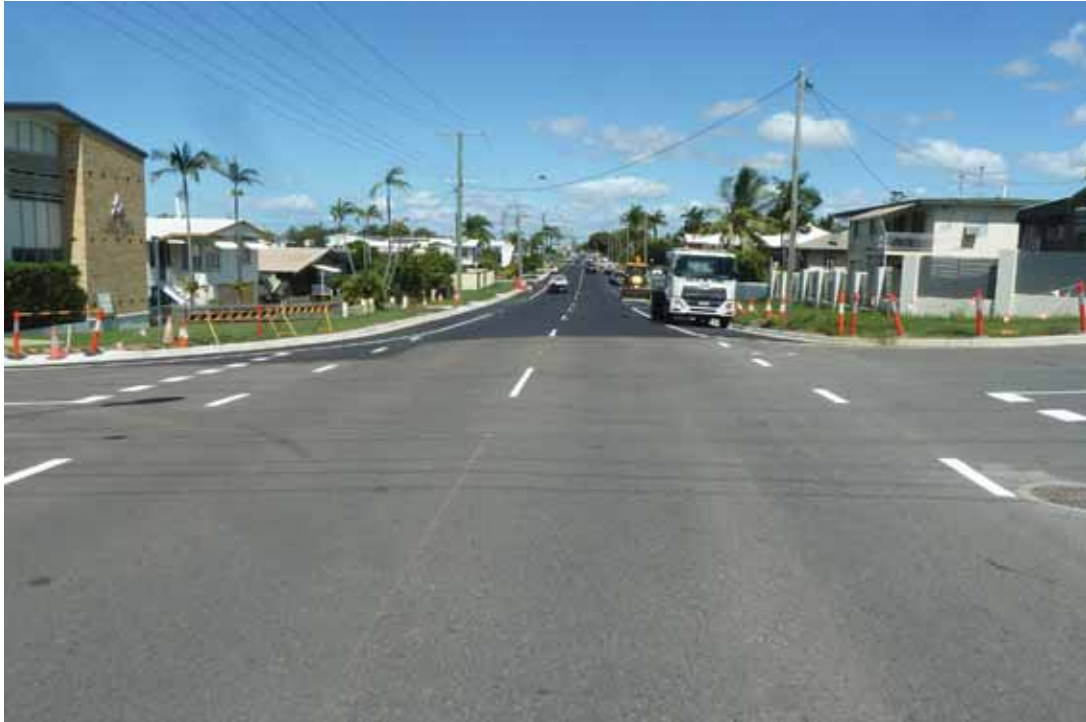
Gladstone-Toolooa Street - Section 2 of works
