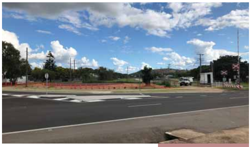
Victory Street-Millchester Road - after
