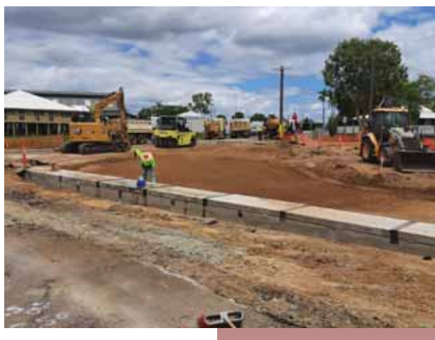
Victory Street - Millchester Road - during
