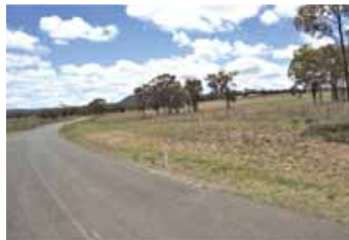
Jack Smith Gully Road – before
