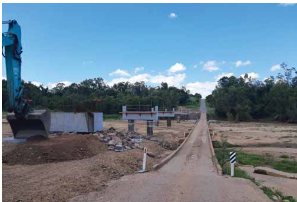
Ted Cunningham Bridge - construction underway
