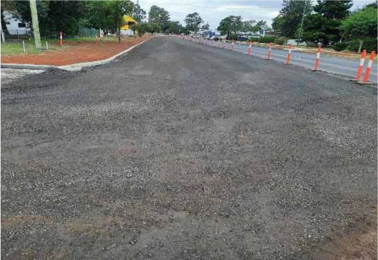
Glasson Street - nearing completion
