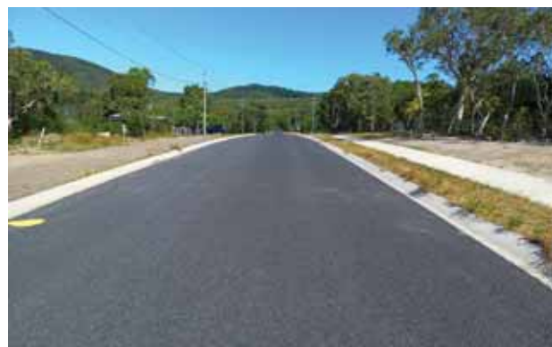
Sealed Garden Street, including footpath and ancilliary drainage
