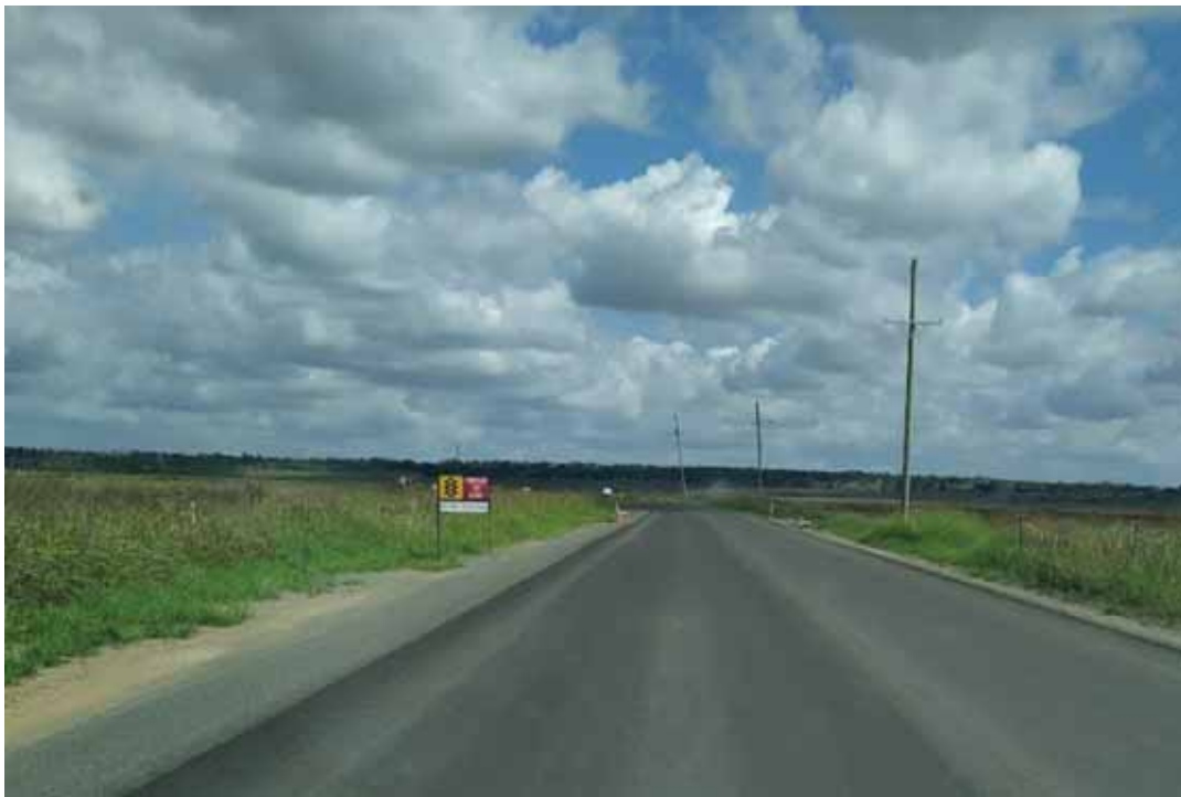
Sealed portion of road (Primerseal) from Ch410 - Ch1245
