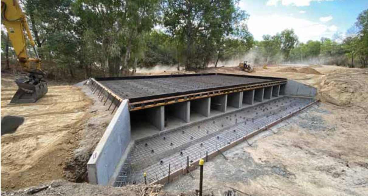
Magnificent Creek Overflow - during
