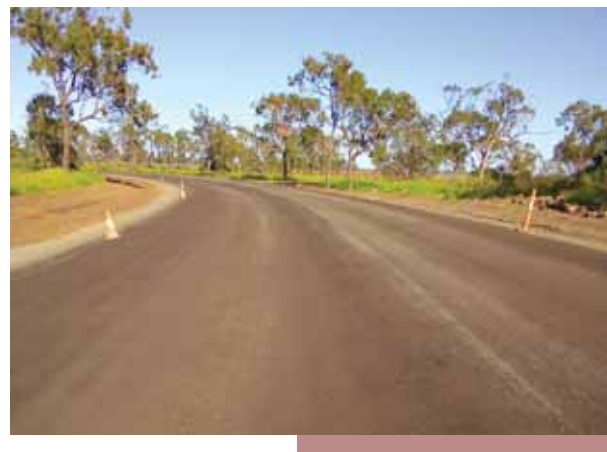
Unbound pavement ready for seal
