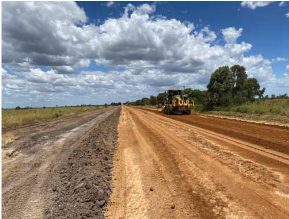
Valkyrie Road upgrade - during
