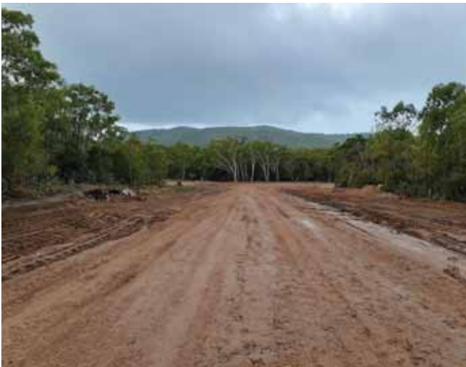
Subgrade preparation, Garden Street
