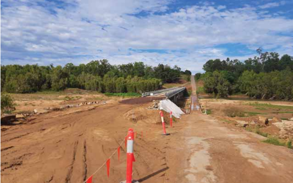
Ted Cunningham Bridge - nearing completion
