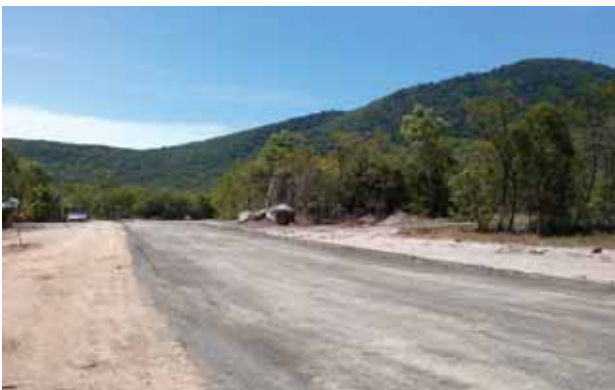
Pavement construction, Boundary Street
