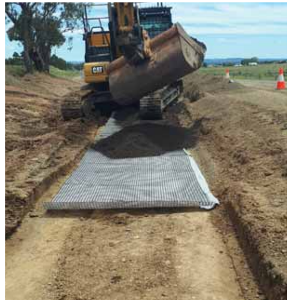
Jack Smith Gully Road - geofabric
