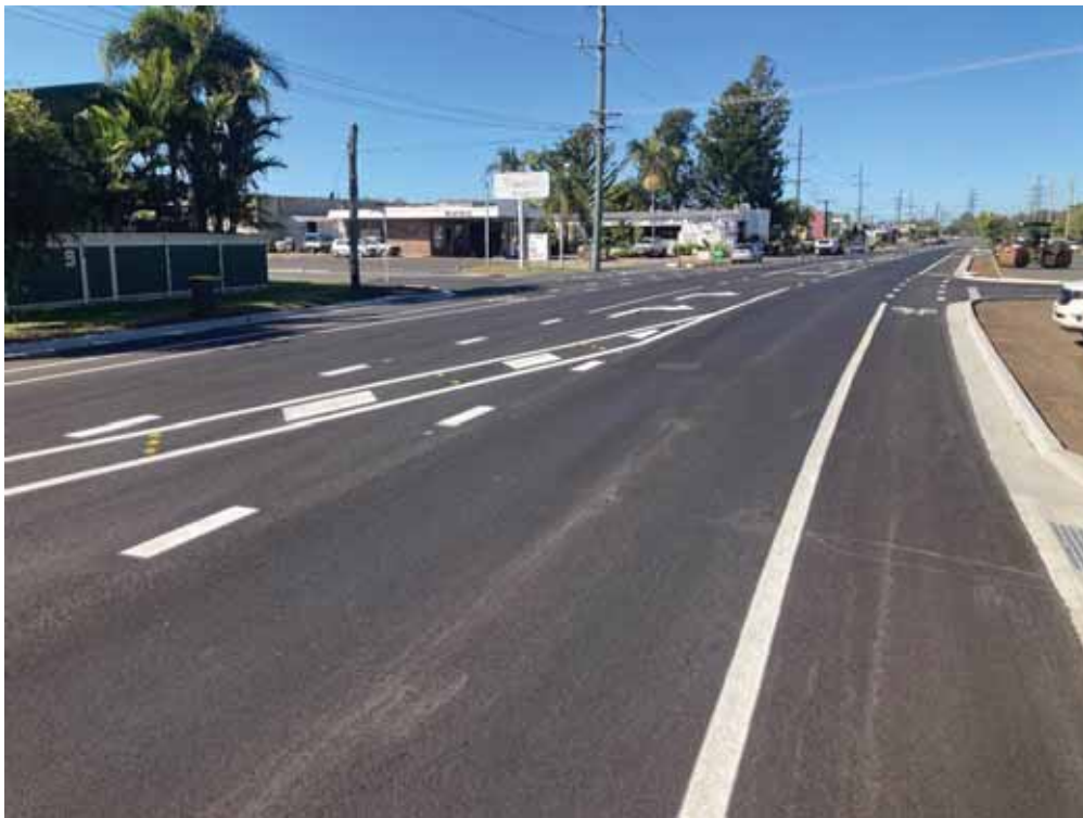
Glenmore Road & Park Road intersection - completed
