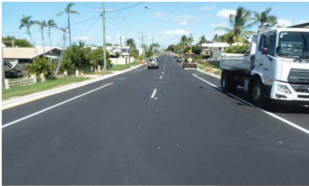
Gladstone-Toolooa Street - view south of the full extent of works
