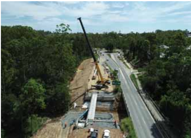
Springfield Greenbank Arterial Road and Springfield Parkway - upgrade bridge beams
