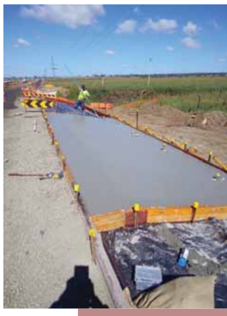
Batter protection under construction
