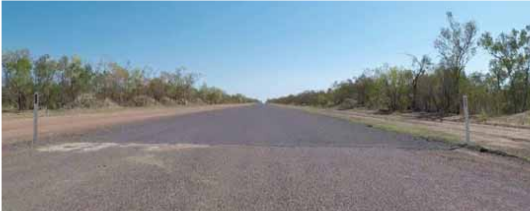
Richmond-Croydon Road - after (Ch 126)
