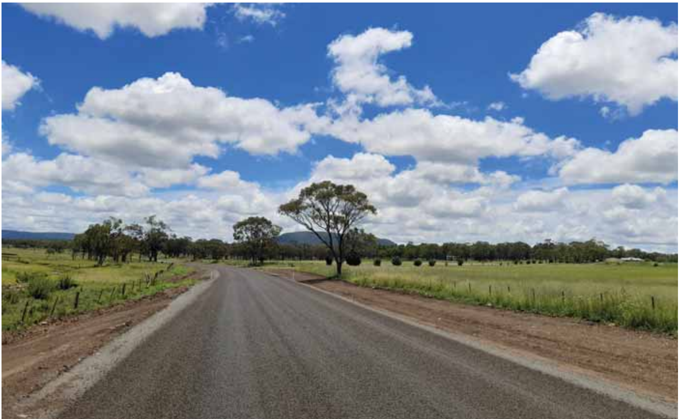
Jack Smith Gully Road - completed
