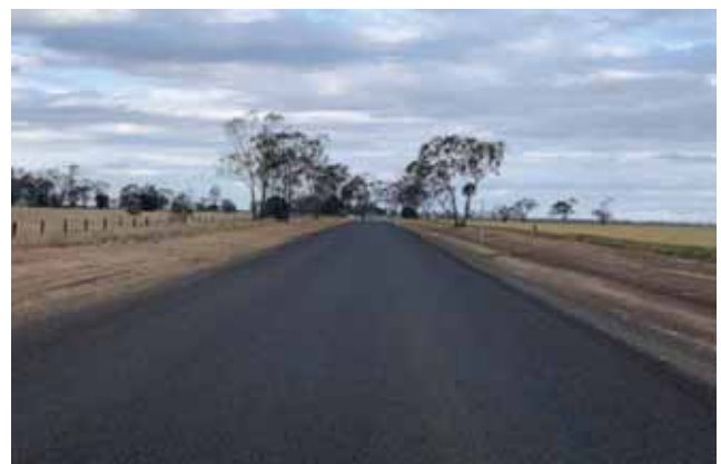
Wilds Road – after
