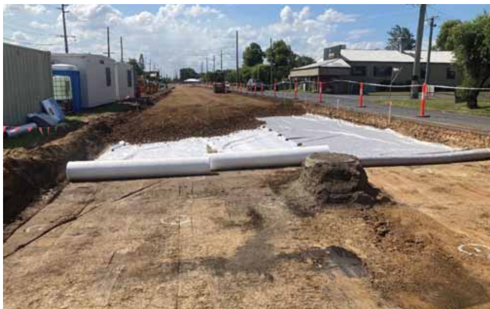
Glenmore Road - subgrade and placement of subbase layer on geofabric
