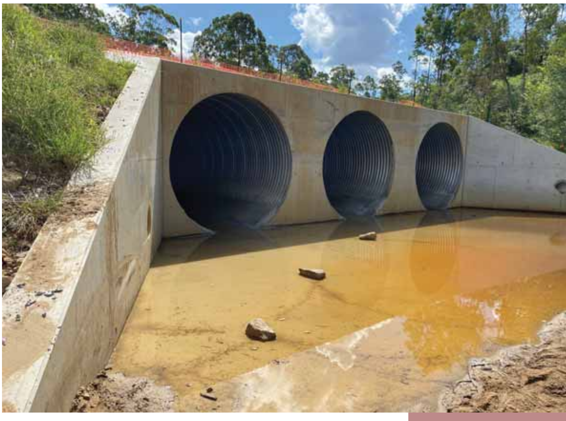
Springfield Greenbank Arterial Road and Springfield Parkway - 3.6m culverts with lining
