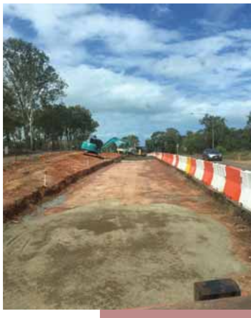
Rockhampton-Tarangba Road - construction
