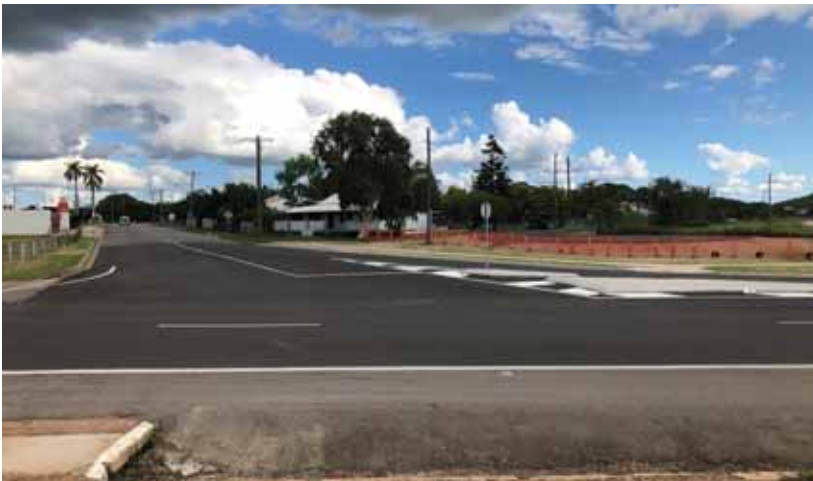
Victory Street-Millchester Road - after
