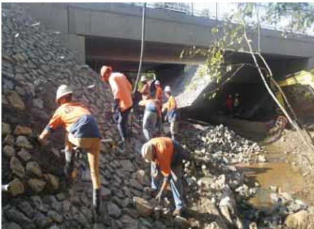
Springfield Greenbank Arterial Road and Springfield Parkway - upgrade bridge rock protection
