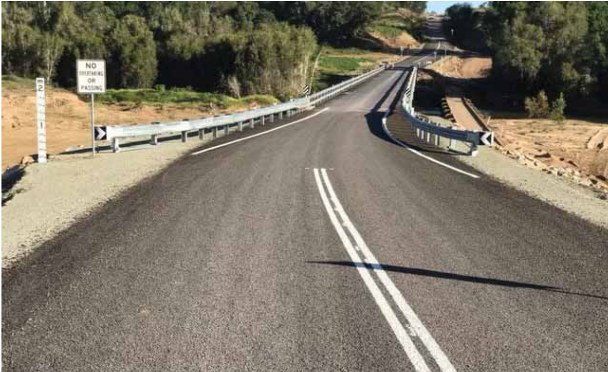
Ted Cunningham Bridge - completed
