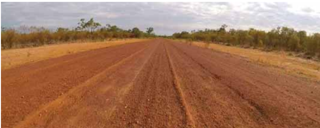
Richmond-Croydon Road - before (Ch 138)
