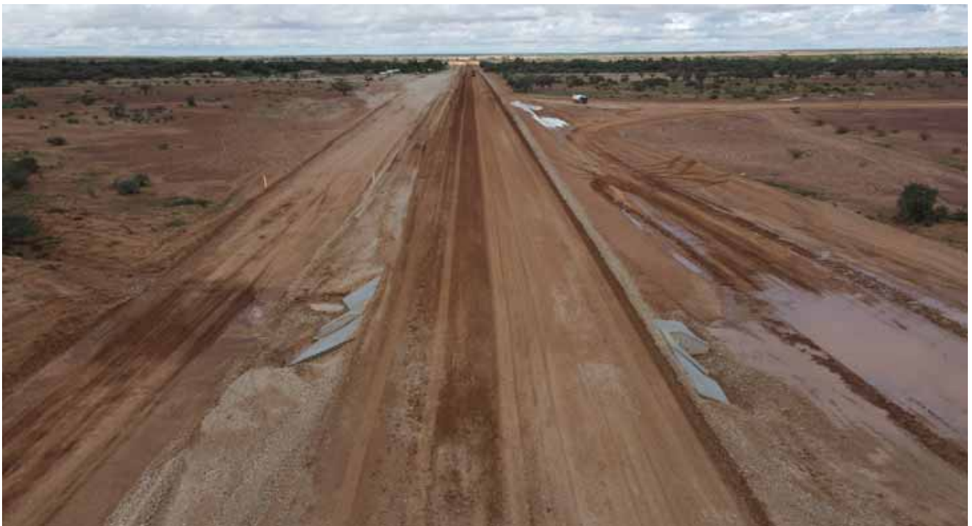
Bedourie-Birdsville - culvert installation
