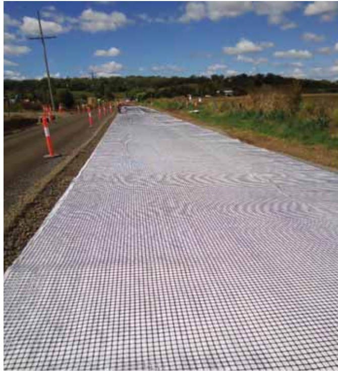
Installation of high-strength synthetic material
