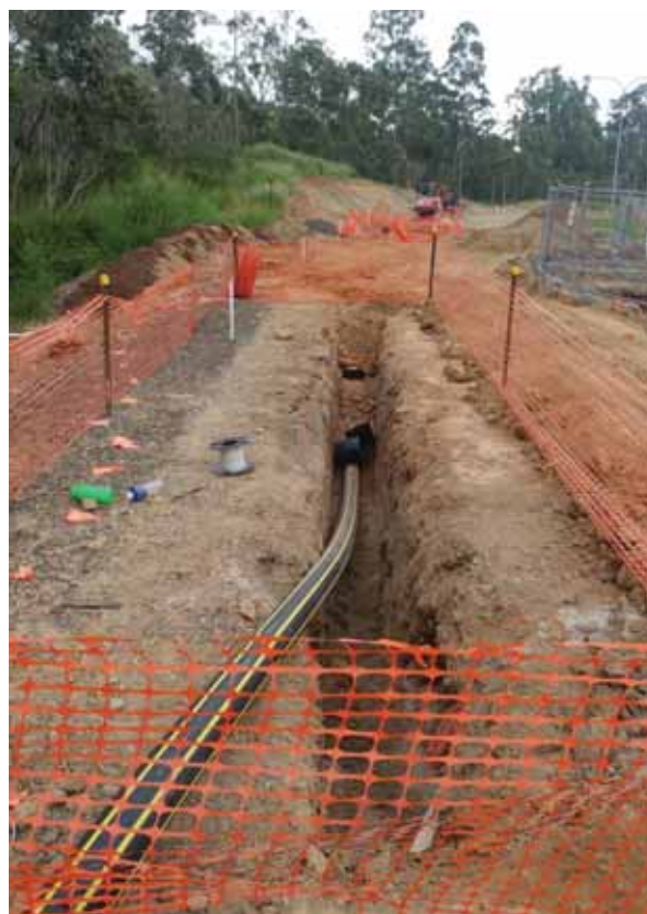
Springfield Greenbank Arterial Road and Springfield Parkway - APA Gas
