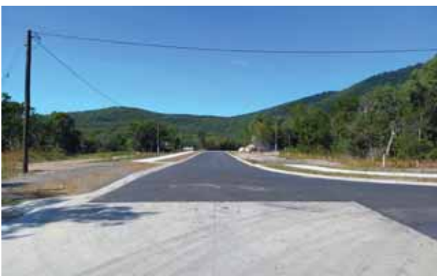
Sealed Boundary Street, including footpath and ancilliary drainage
