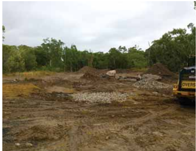
Unsuitable material replacement (Garden Street and Boundary Street Intersection)
