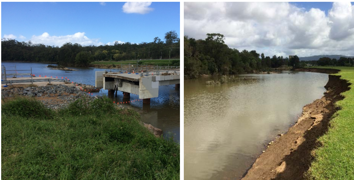
Figure 5.2.6.1 – Bridge in South East Queensland
