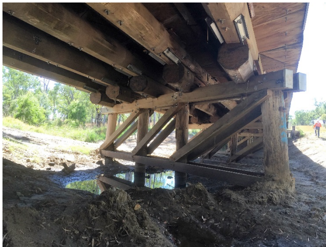
Figure 5.4.12(h) – Existing Doubtful Creek Bridge (looking downstream)
