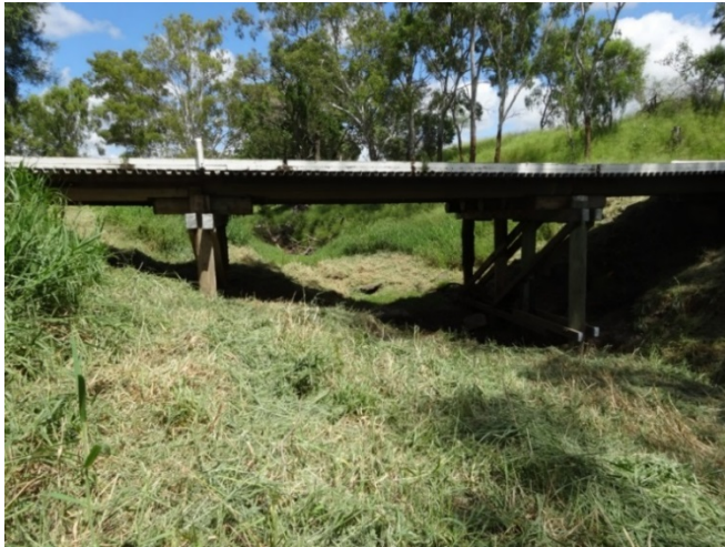
Figure 5.4.12(c) – Existing North Kariboe Creek Bridge (looking downstream)
