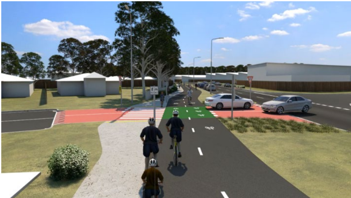
Figure 4.3(b) – Example of two-way cycle track, 5 m buffer from the carriageway at raised priority crossings (LTS1)
