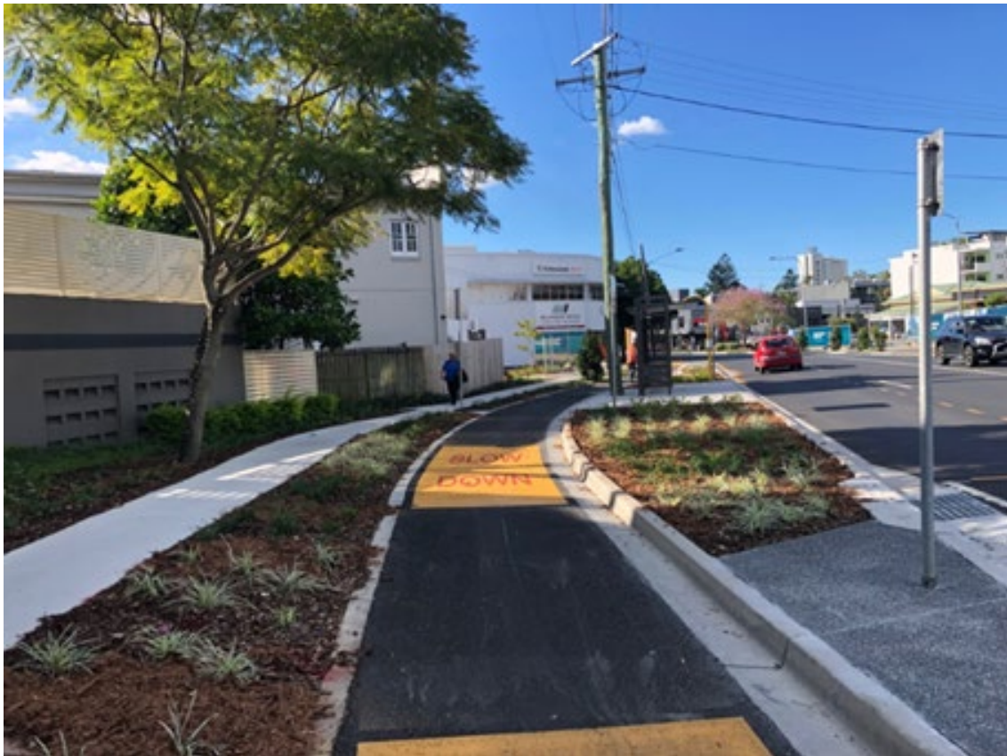
Figure 3.3.3(b) – One-way cycle track behind bus stop, Annerley Road, Brisbane
