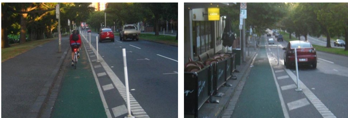
Figure 3.2.5 – Buffered bicycle lane with clearway during peak hour and car parking in off-peak, Albert Street, Melbourne
