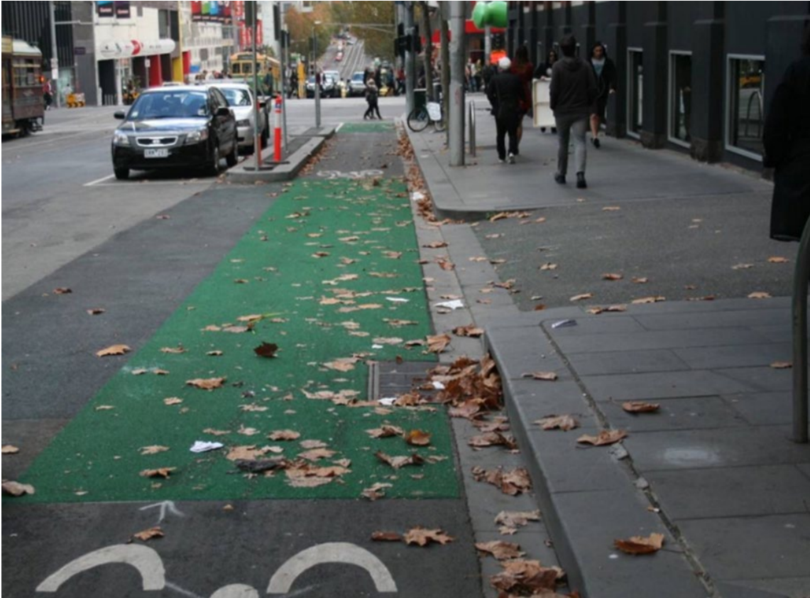
Figure 3.2.1(c) – One-way cycle track under construction, Latrobe Street, Melbourne
