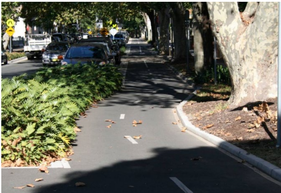
Figure 3.3.2 – Two-way cycle track diverted around existing street tree, Bourke Street, Sydney
