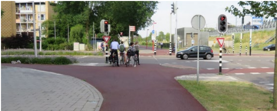
Figure 4.5.2(a) – Three-aspect lanterns for bicycle traffic at low and high heights at nearside
