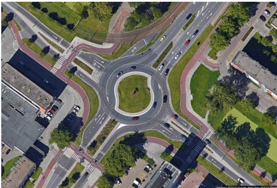
Figure 4.4.2(a) – Multiple lane roundabout with single lane priority crossings, Utrecht (LTS1)
