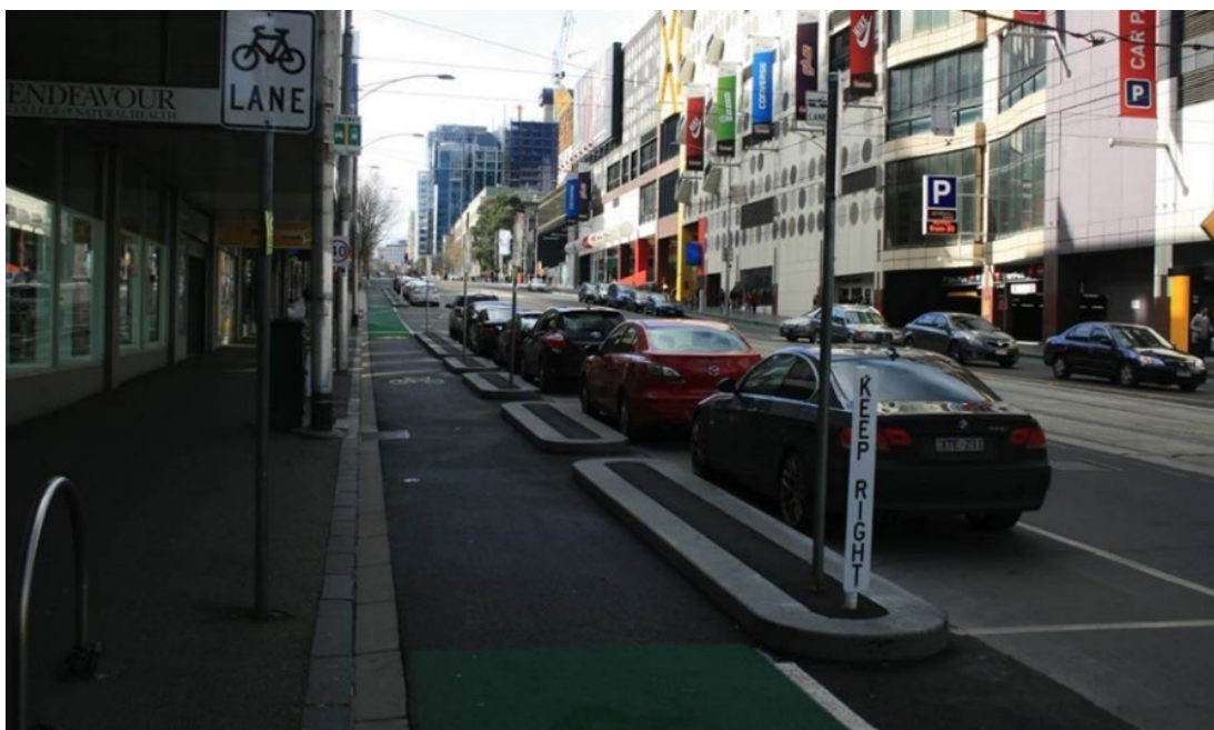
Figure 3.2.1(a) – One-way cycle track, Latrobe Street, Melbourne
