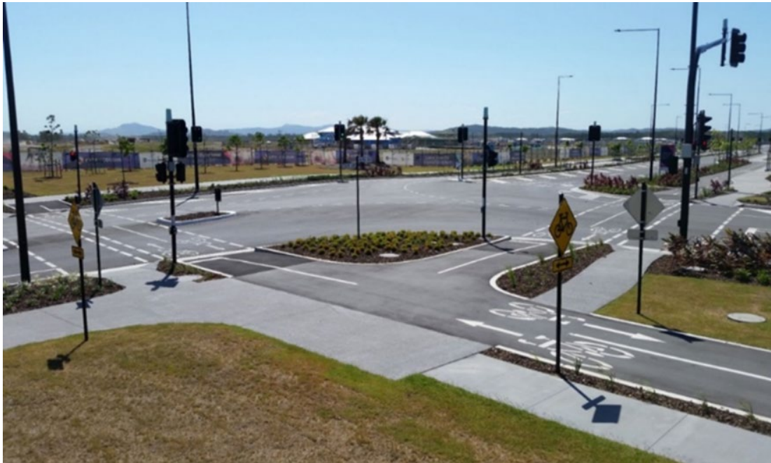
Figure 4.5(a) – Protected signalised intersection with two-way cycle tracks, Aura Boulevard / Central Avenue, Nirimba
