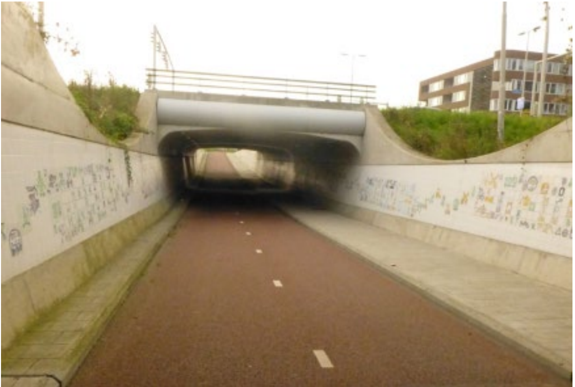
Figure 4.6(b) – Pedestrian and bicycle underpass with artwork created by local primary school children, Nijmegen, Netherlands
