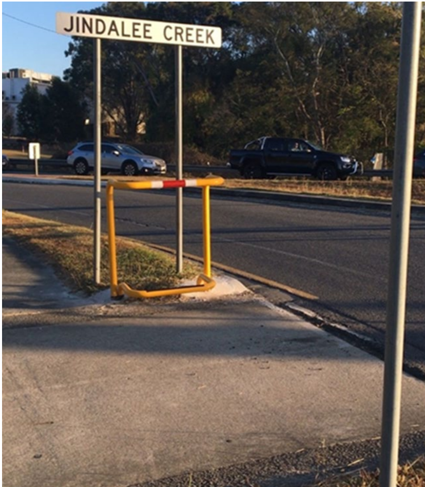
Figure 4.5.1(h) – Holding rails and foot rails for comfortable waiting at signalised crossing, Jindalee
