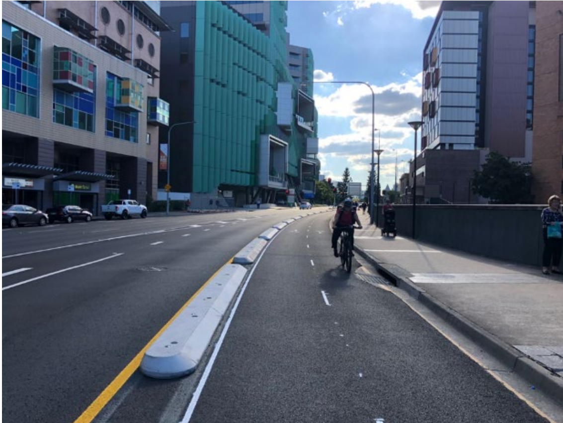
Figure 3.2.6.2(a) – Two-way cycle track, median separated profile, Stanley Street, South Brisbane
