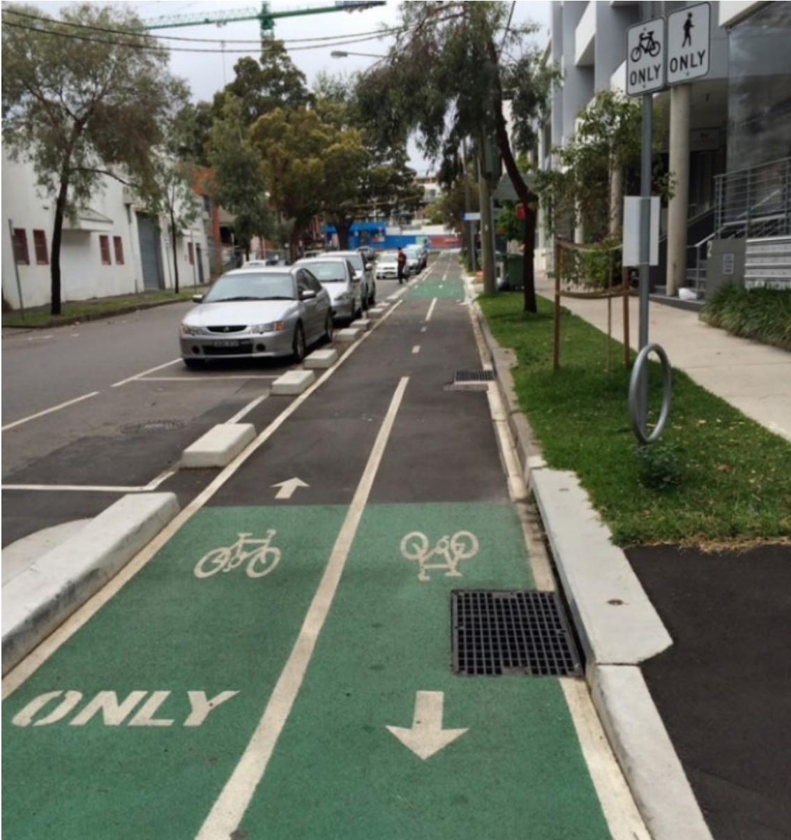
Figure 3.2.1.1(b) – Two-way cycle track and parking, Sydney
