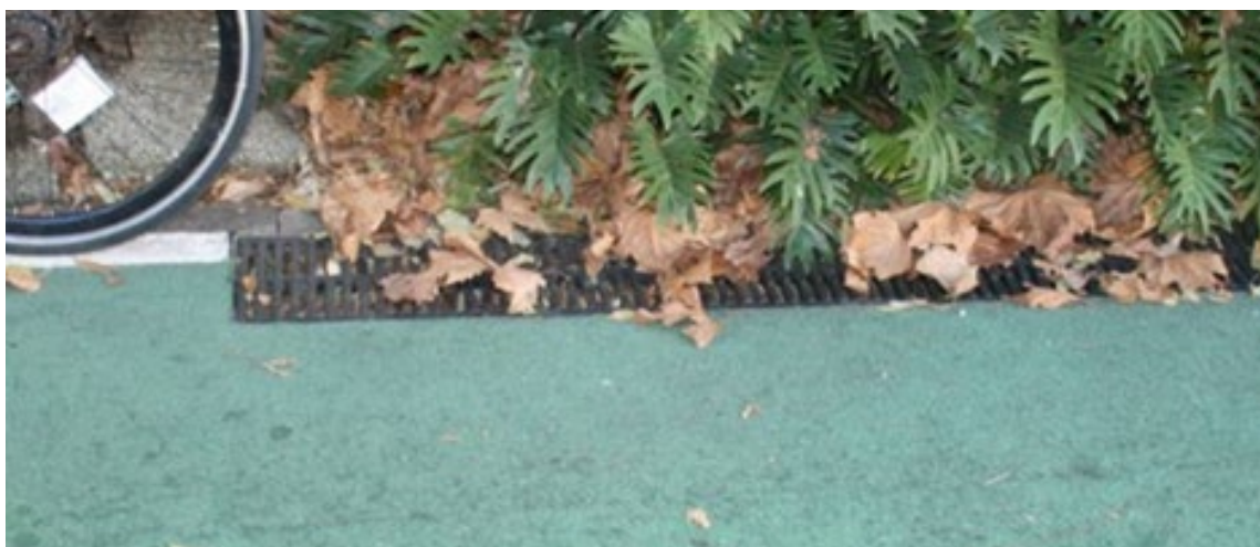
Figure 3.2.6.3(d) – Two-way cycle track at footpath level with drain alongside planting strip, Bourke Street, Sydney
