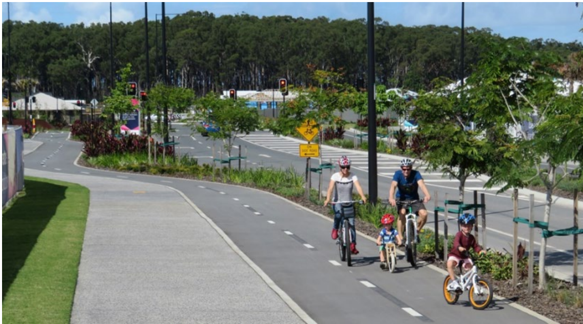
Figure 3.2.2(a) – Two-way cycle track mid-block in a new development, Aura, Caloundra
