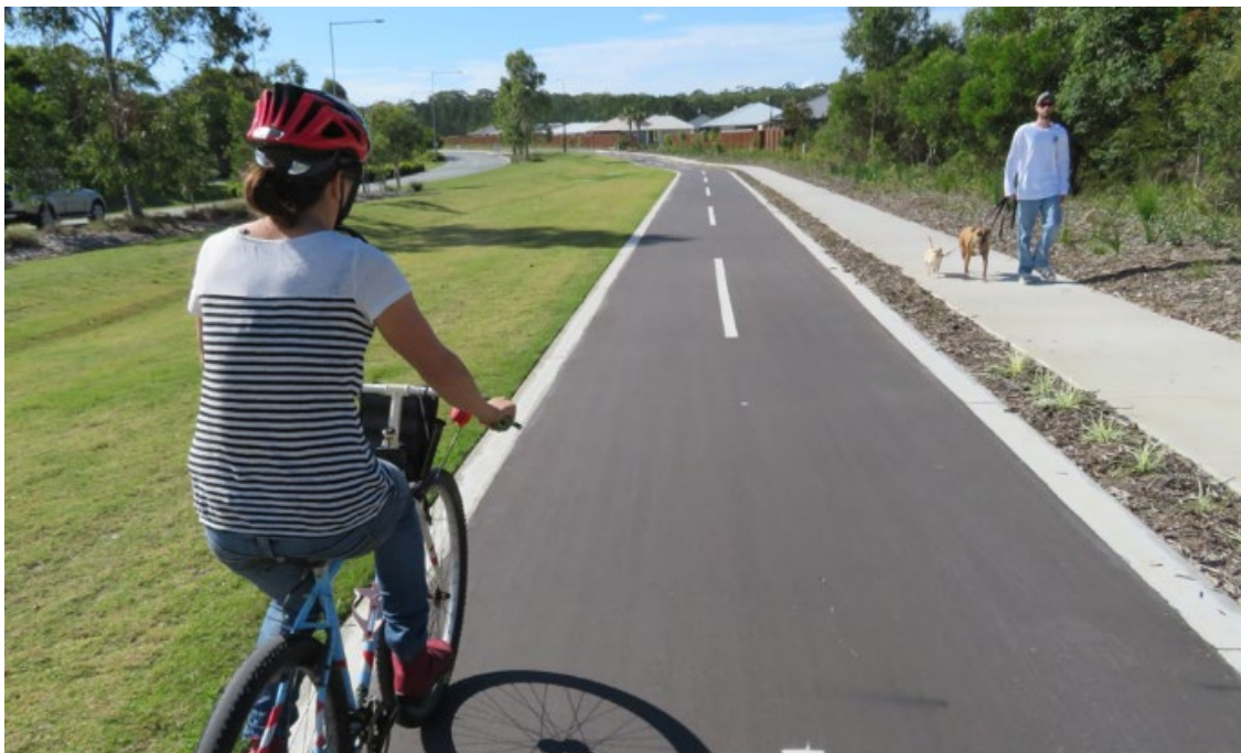
Figure 3.2.6.3(b) – Two-way cycle track – planting separation, Aura, Caloundra
