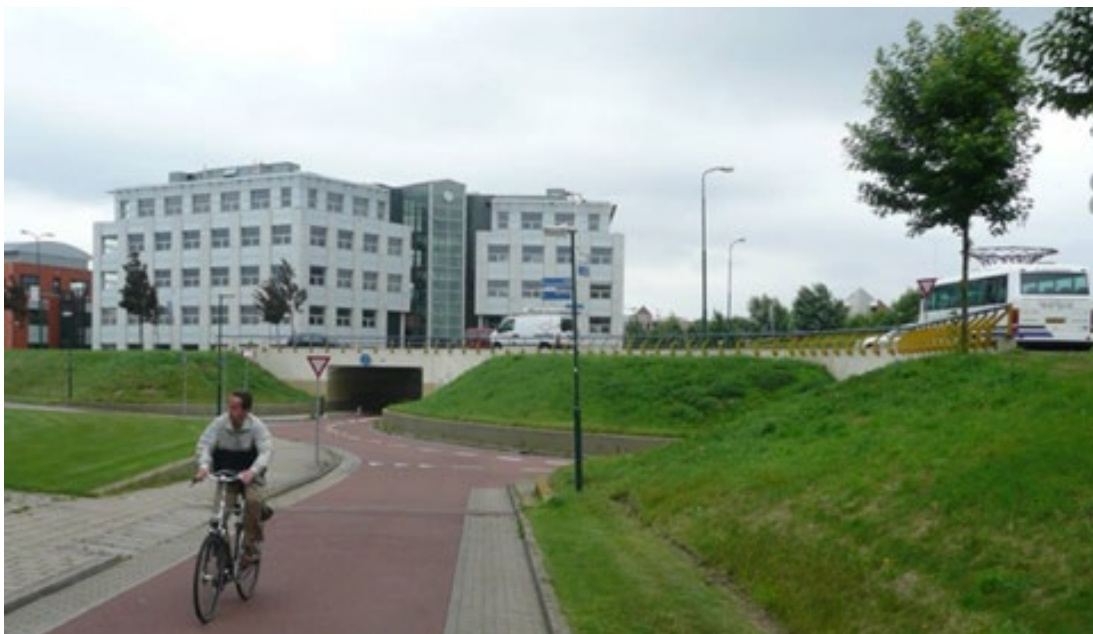
Figure 4.4.2(c) – Grade-separated roundabout, Houten, Netherlands (LTS1)
