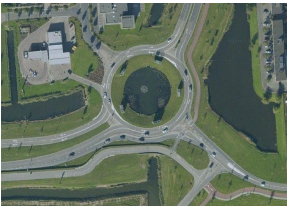
Figure 4.4.3 – Urban multiple lane roundabout, Rotterdam, Netherlands (LTS2)
