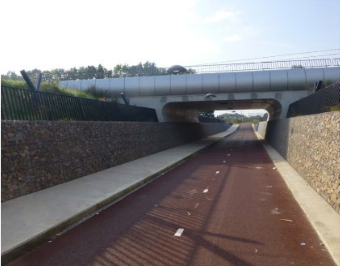
Figure 4.6(a) – Pedestrian and bicycle underpass with rock walls, Nijmegen, Netherlands
