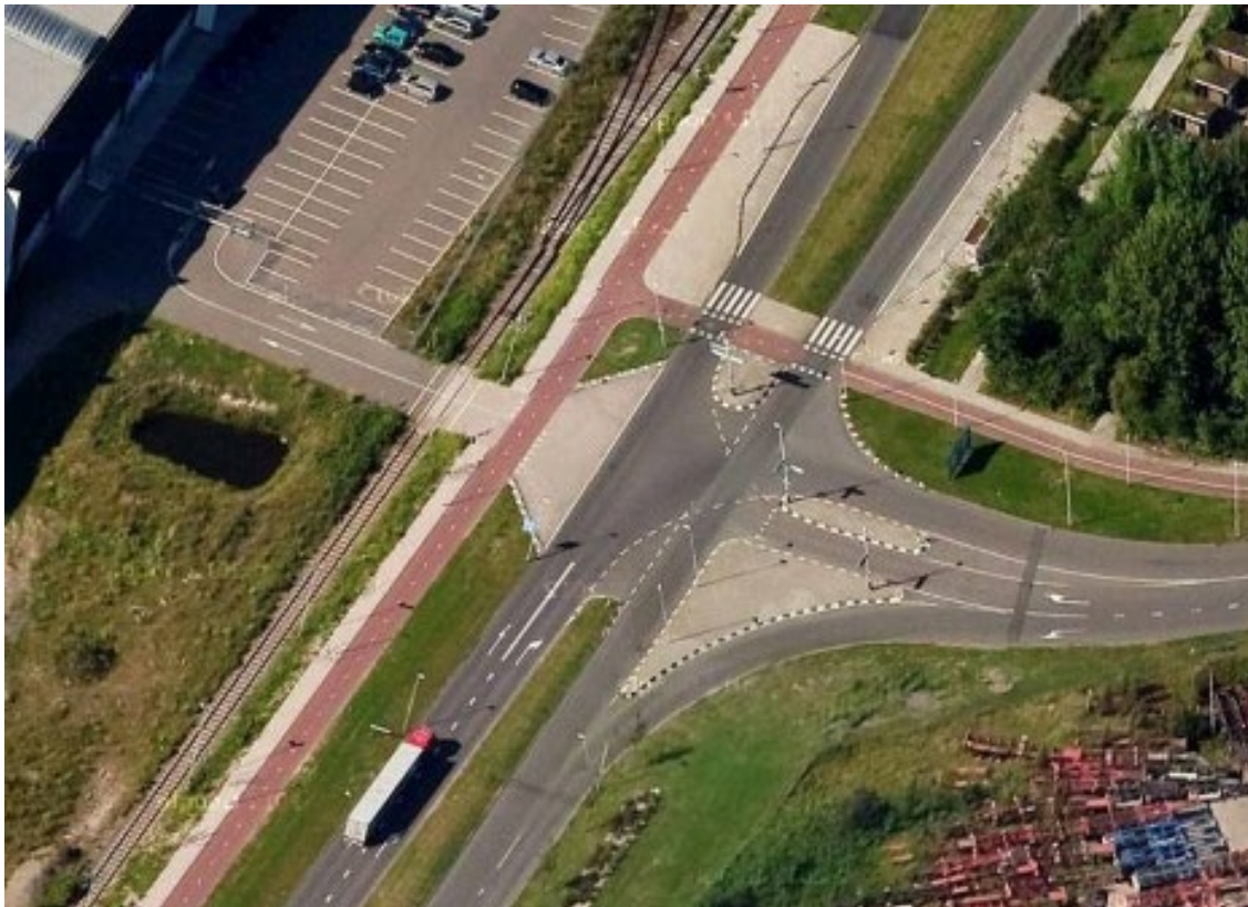
Figure 4.7.2 – Two-way cycle track crossing industrial area driveway, Rotterdam
