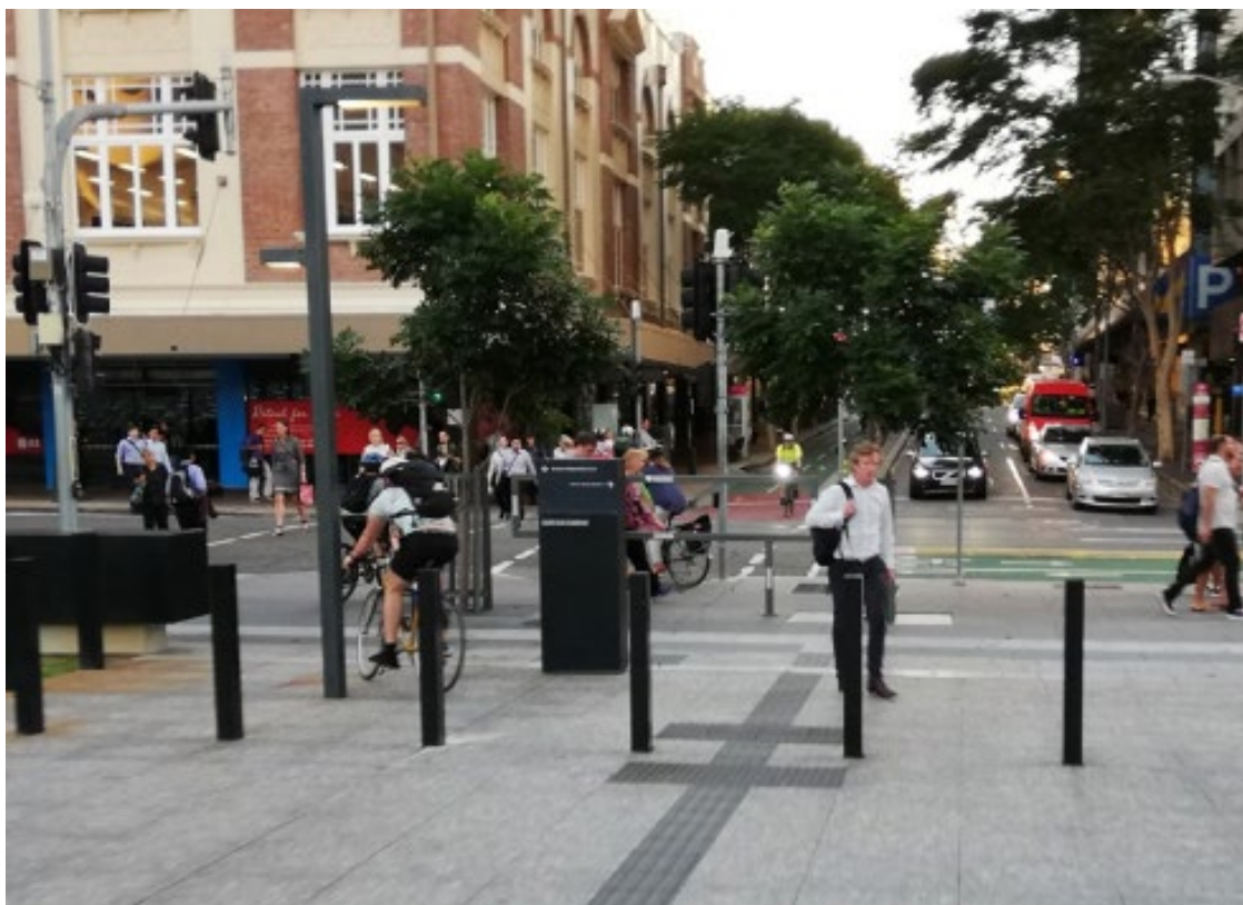
Figure 4.5.1(g) – Hazard blocking the movement of people cycling and walking resulting in conflicts
