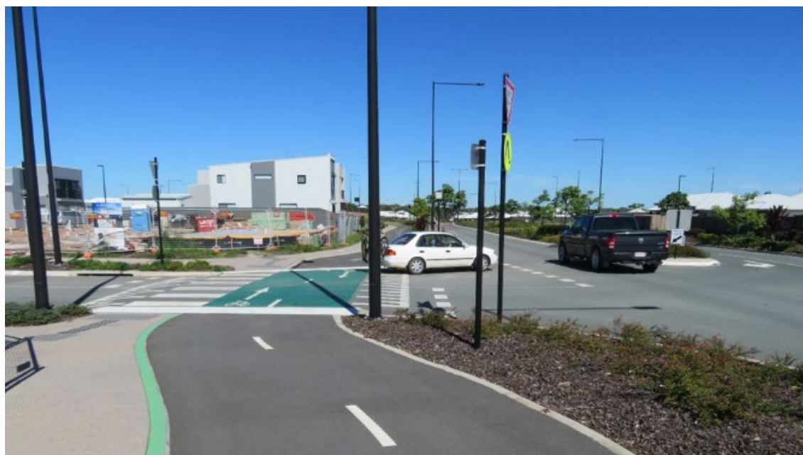
Figure 4.3(a) – Protected unsignalised intersection with two-way cycle track and separate footpath with zebra pedestrian crossing, Aura, Caloundra (LTS1)
