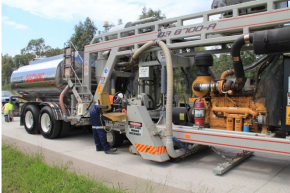
Figure 7(h) – Diamond grinding in progress
