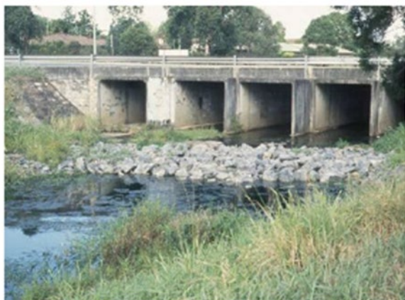
Figure 3.9 – Box Culverts with riprap
