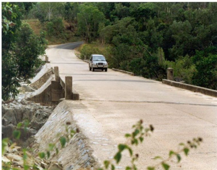
Figure 4.1 – Little Annan River floodway crossing
