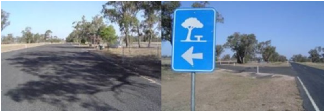
Figure 6B-10 – Rural rest area 14 km north of Surat on Carnarvon Highway provides shade, shelter, table and water
