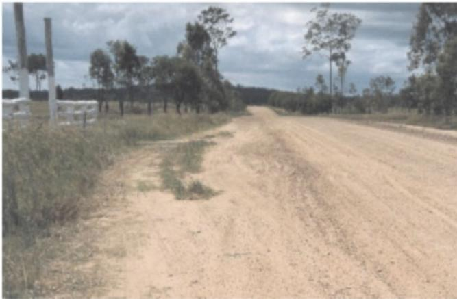
Bus stopping area is unsatisfactory due to poor skid resistance during wet weather conditions.
