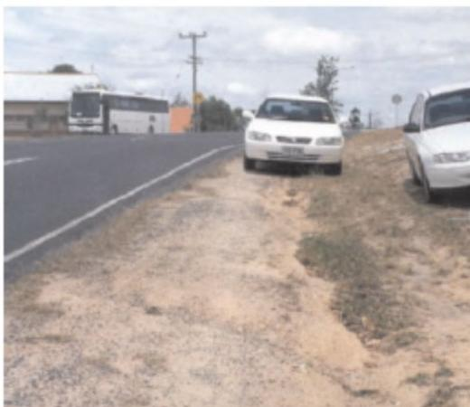
There is inadequate width for the school bus to be positioned completely clear of the travel lane.
