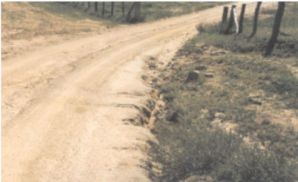
Pavement appears to be soft with pavement edges deeply scoured. The poor condition of the pavement may be hazardous to the school bus operator and school children as there is a risk of reduced controllability of the school bus.
