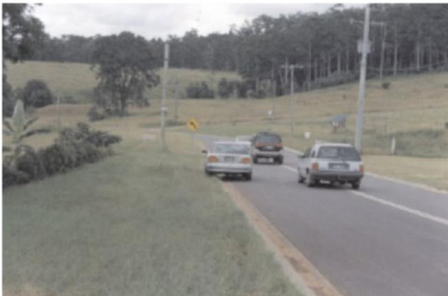
A school bus stop is located where the sedan is parked. There is restricted width between the barrier lines and the kerb (i.e., three metres between parked school bus and barrier lines would not be available as stipulated by legislation). As a result, motorists are forced to cross the barrier lines to pass the parked vehicle. This is illegal and extremely unsafe.
