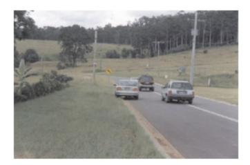
A school bus stop is located where the sedan is parked. There is restricted width between the barrier lines and the kerb (i.e., three metres between parked school bus and barrier lines would not available as stipulated by legislation). As a result, motorists are forced to cross the barrier lines to pass the parked vehicle. This is illegal and extremely unsafe.
