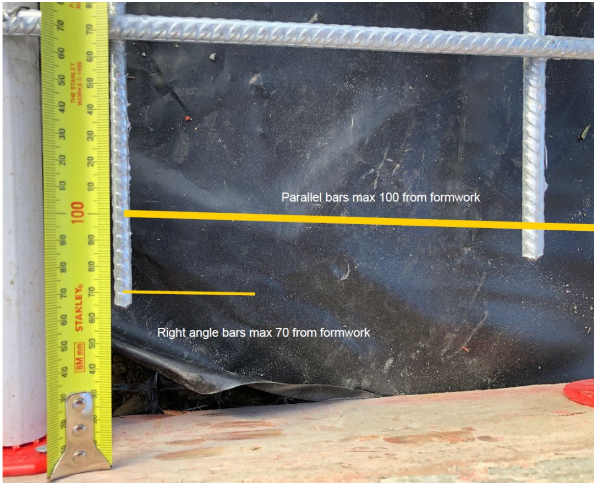
Figure 11.5.3 – Concrete cover requirements
