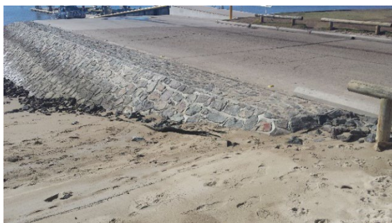
Figure 13.5 – Examples of acceptable grouted rock shoulder construction
