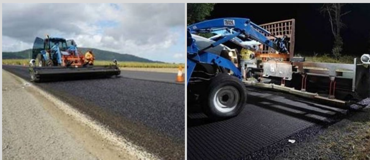
Figure 9.6.2 – Installation of asphalt geosynthetics using application frame attached to a tractor
