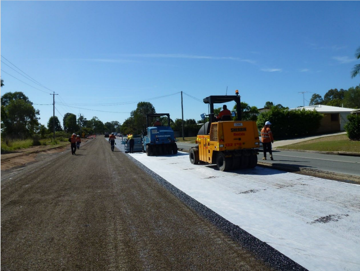
Figure 8.7.2(b) – Geotextile installed using application frame attached to multi-tyred roller
