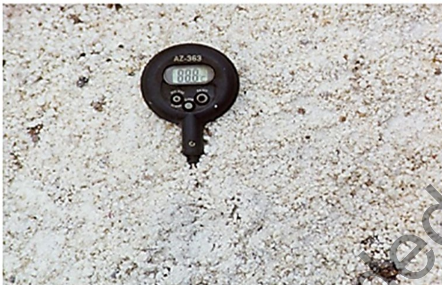
Figure 8.6.5.3 – Checking completion of slaking with temperature probe
