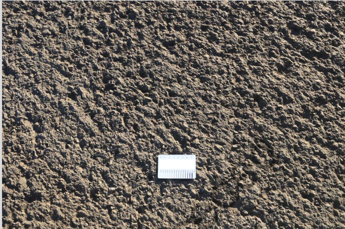
Figure 8.9.9.4(b) – Example of an acceptable hard-cut surface
