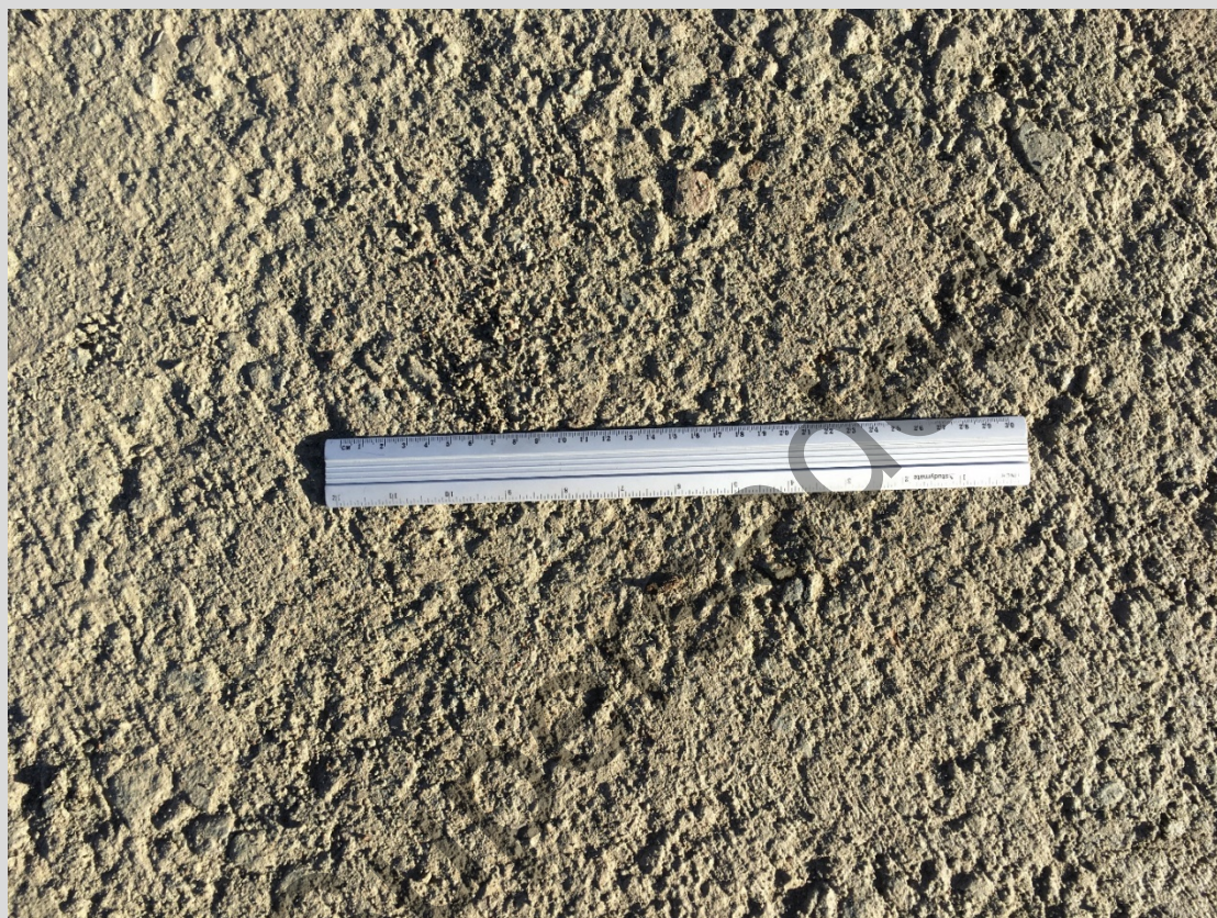
Figure 8.2.8.2 – Example of acceptable cut-back surface
