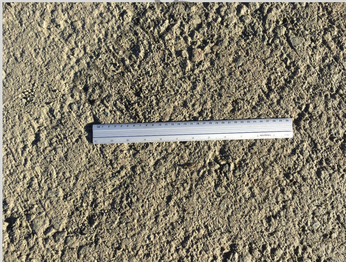
Figure 8.2.7.2 – Example of acceptable hard-cut surface
