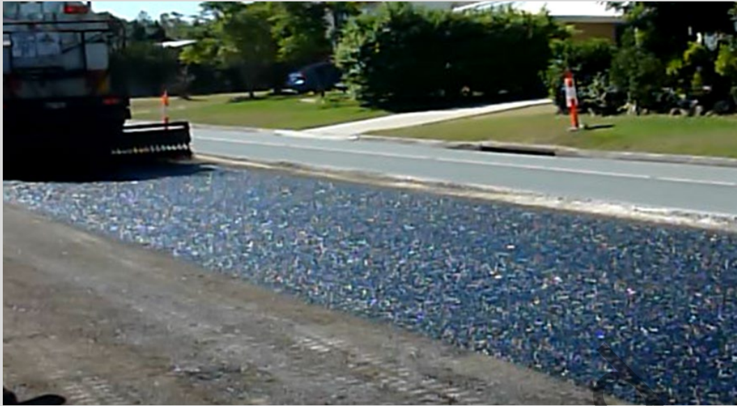
Figure 9.5.3 – C170 bitumen bond coat being sprayed on a prepared pavement surface
