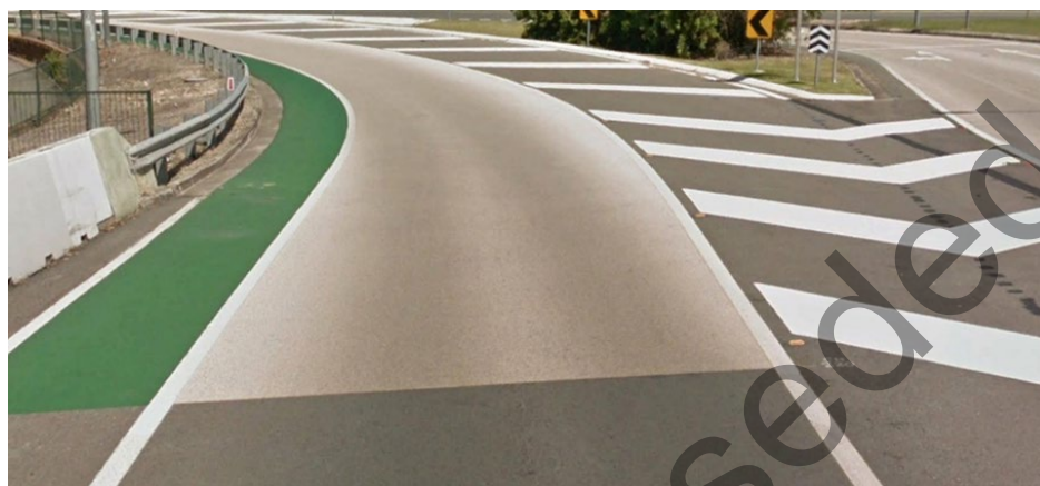
Figure 1 – Typical HFST on a tight curve
