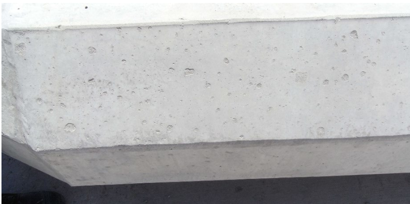
Figure 6(b) – Unacceptable surface finish (Face D)
