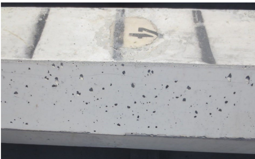
Figure 6(b) – Unacceptable surface finish (Face D)
