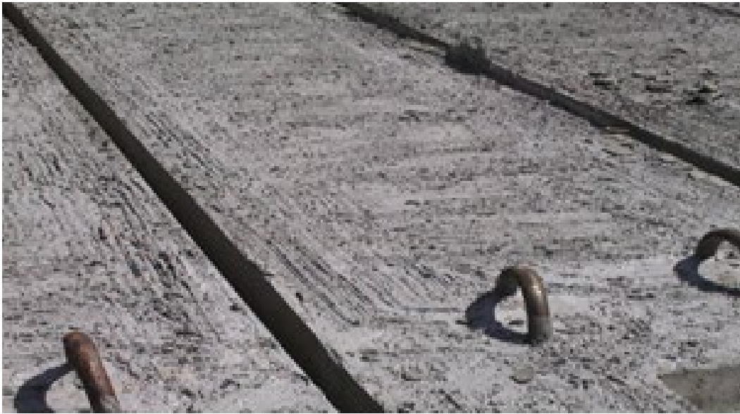
Figure 3 – Acceptable broom finish
