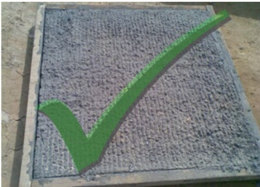
Figure 4(b) – Acceptable raked finish
