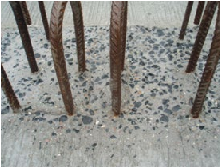
Figure 4(a) – Acceptable construction joint finish
