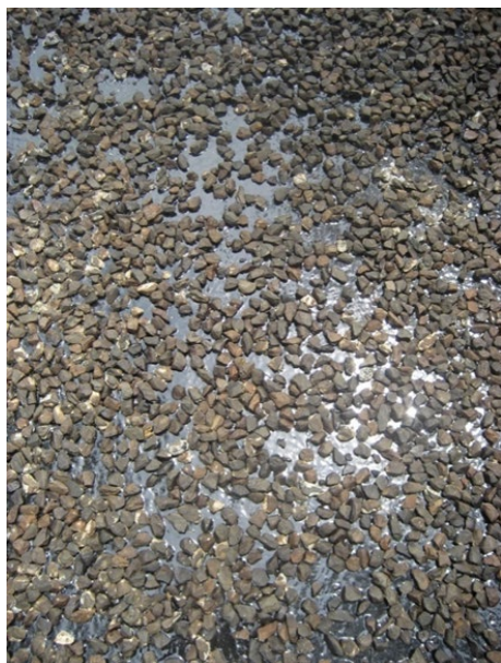
Figure Q6.8.1 – 14 mm aggregate typical appearance prior to multi-tyred rolling
