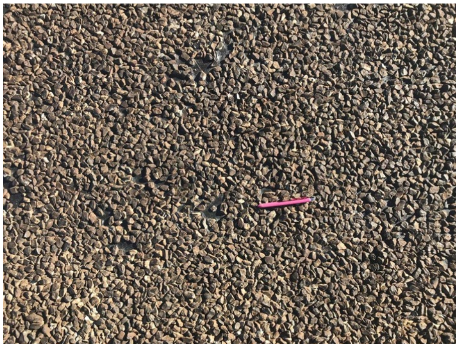
Figures Q6.8.2 and 6.8.3 – 14 mm aggregate typical after multi-tyred rolling
