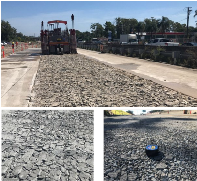
Figure 5.2.2 – Rubblisation works
