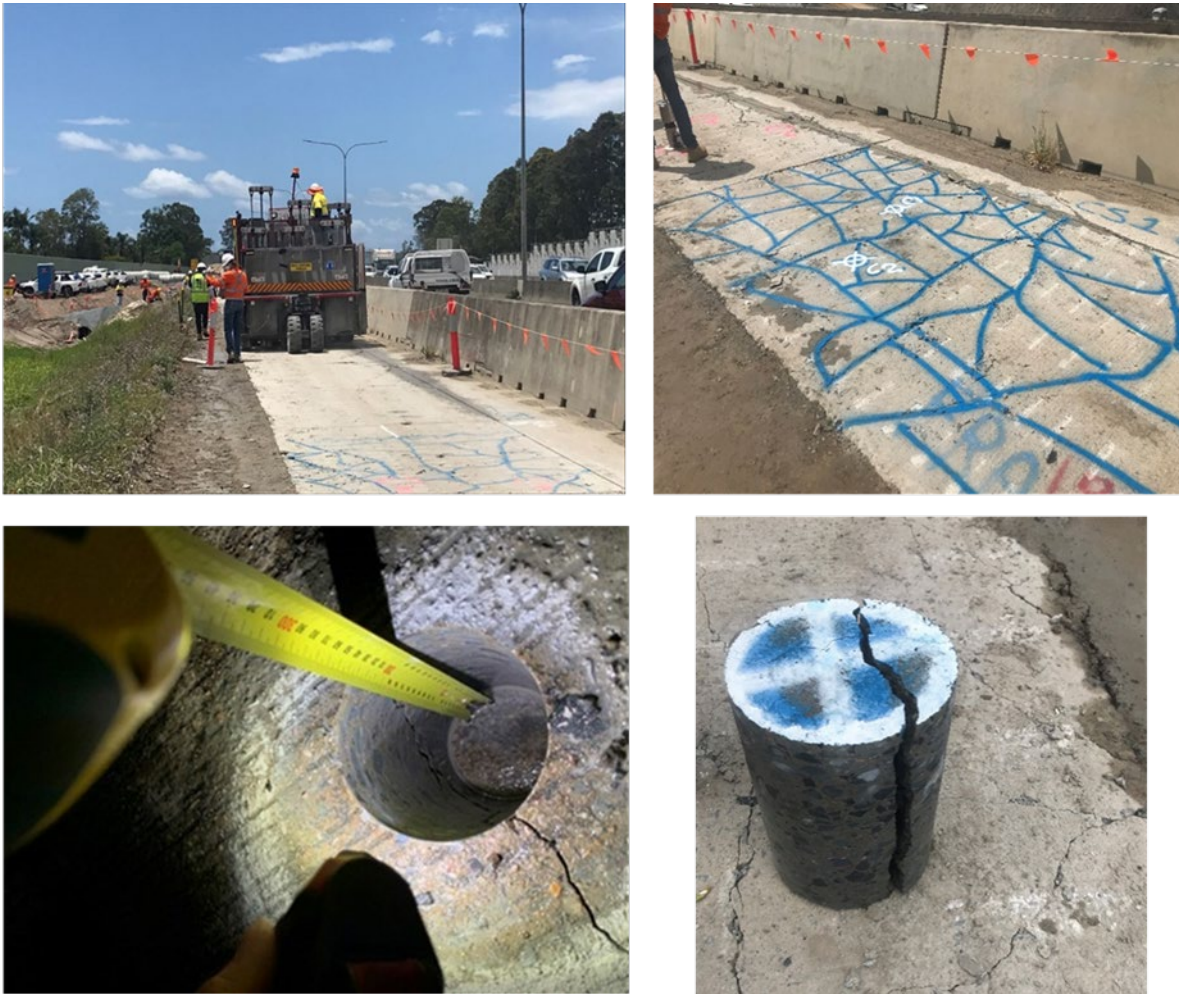
Figure 5.2.3 – Crack and seat works
