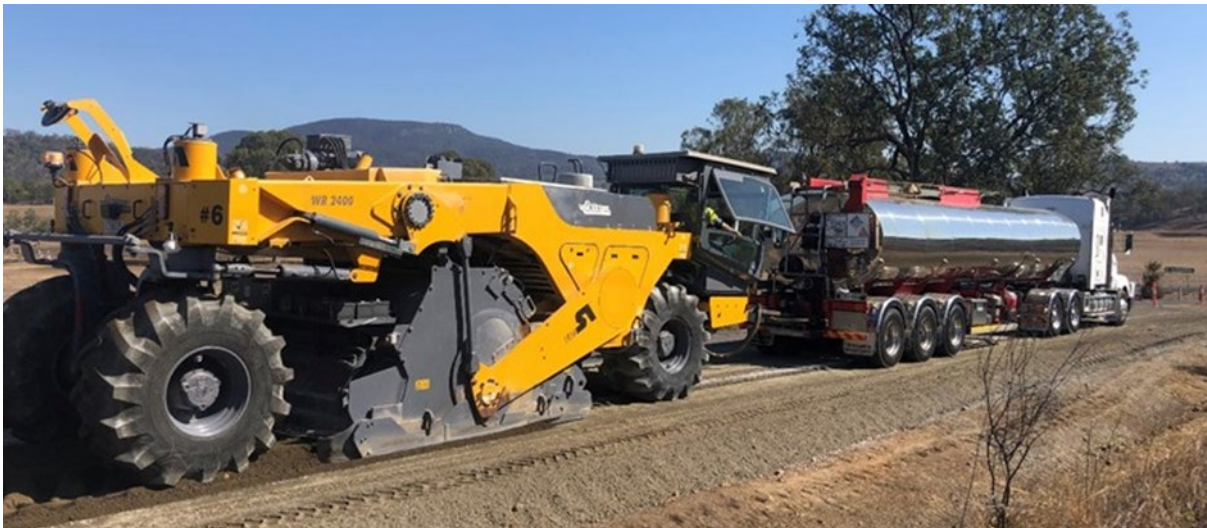
Figure 5.1 – Insitu stabilisation works
