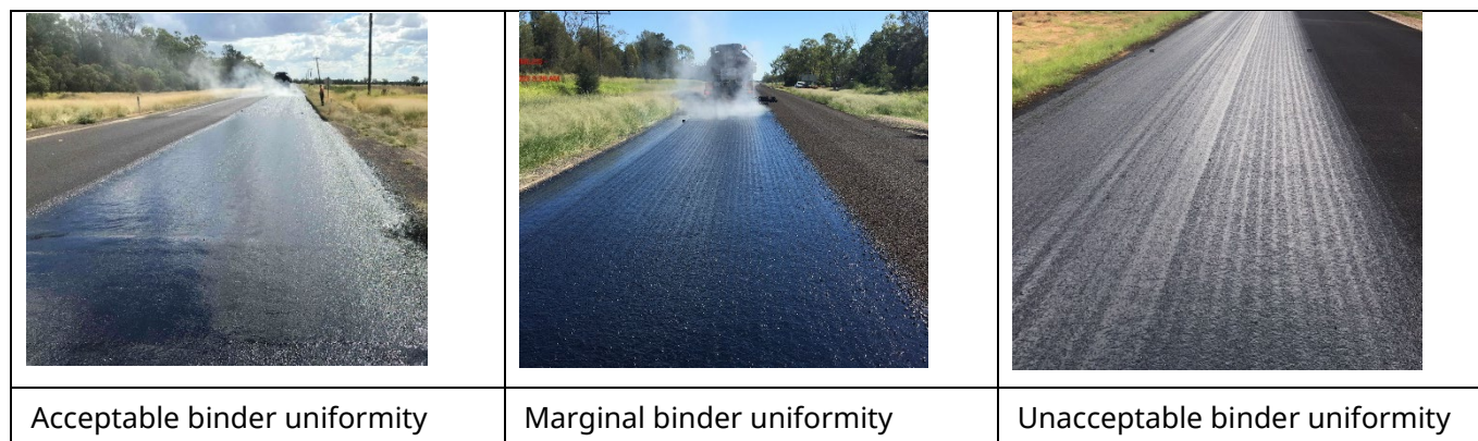
Figure 6.1.2 – Visual examples of binder uniformity
