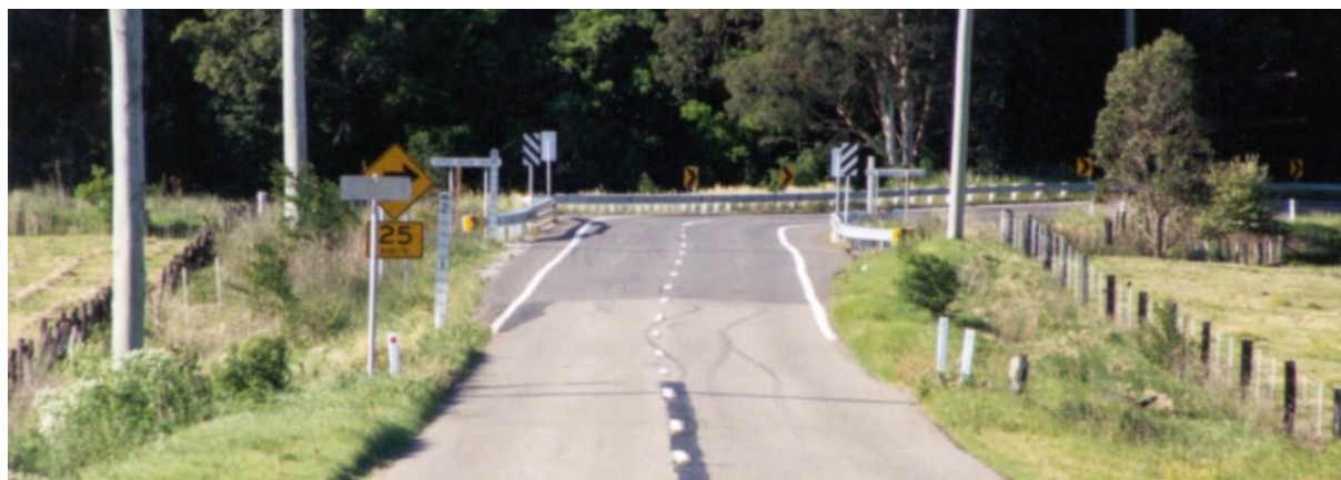
Figure C.8 – Looking north to the reconstructed bridge and curve
