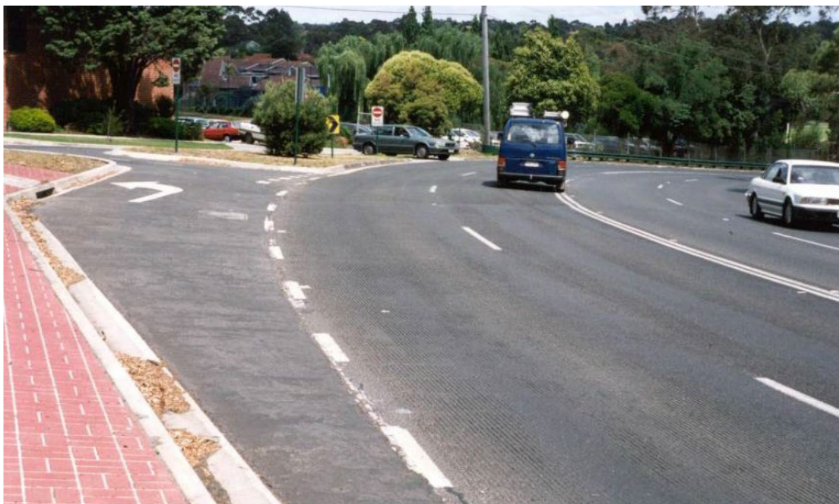
Figure D.6.2 – Inadequate lane width for southbound traffic on the south curve
