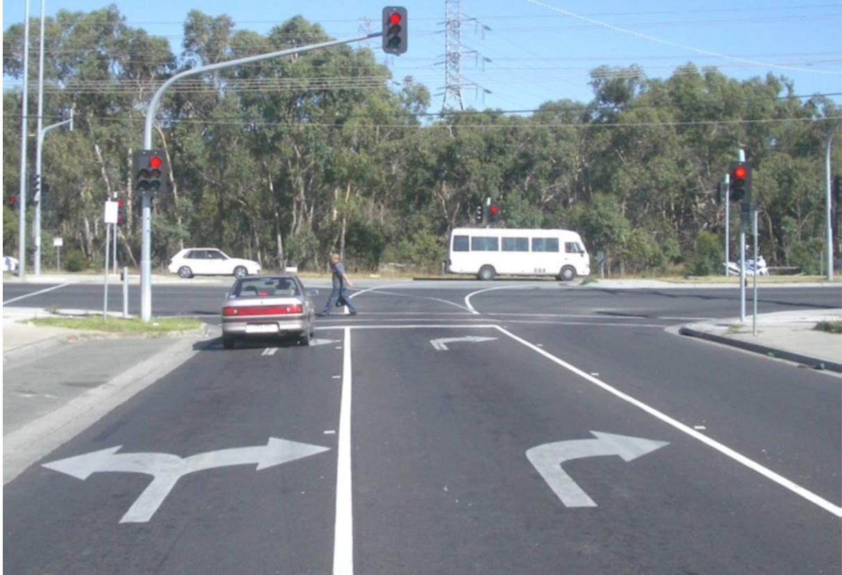
Figure C.7.2 – Example of a recent traffic signal installation
