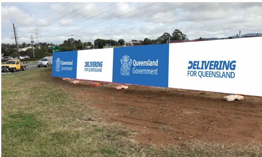
Figure 13.1 – Example of hoarding
