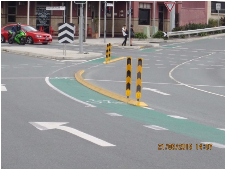
Figure 4.1.3(b) – Gympie Road at Kedron Park Road southbound, Kedron Park (plastic kerb with vertical delineators)
