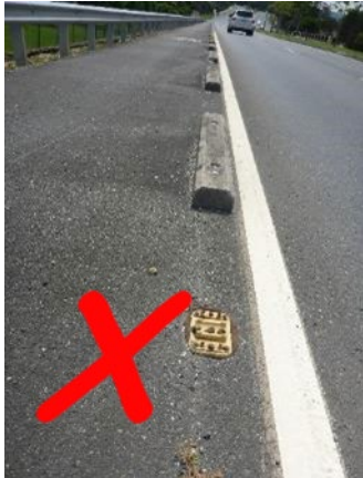
Figure 3 – Example of historical concrete barrier kerbs
