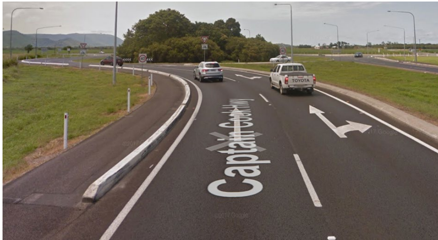
Figure 4.1.2(b) – Captain Cook Highway: current separation treatment (concrete kerb)
