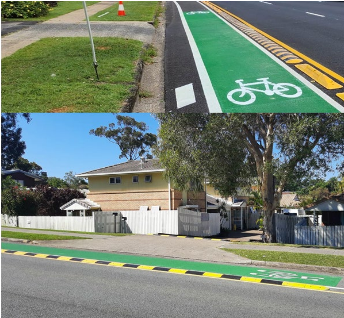
Figure 2.1(b) – Example of traversable (mountable) separation for driveway access
