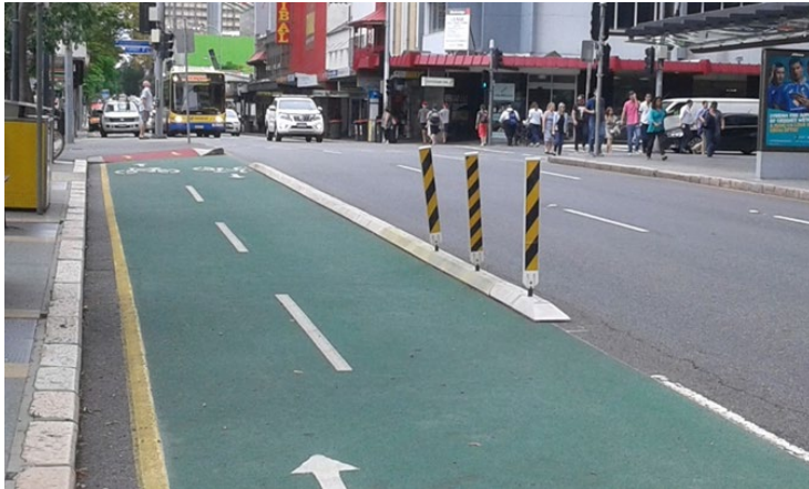
Figure 4.1.3(a) – George Street, Brisbane (plastic kerb with vertical delineators)
