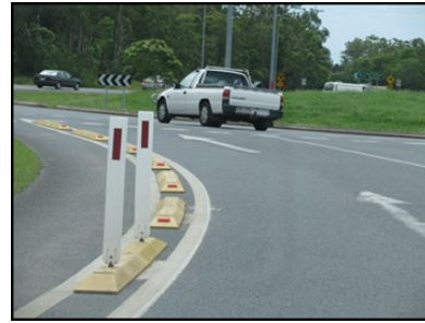
Figure 4.1.2(a) – Captain Cook Highway: 2009 separation treatment (plastic kerb with vertical delineators)
