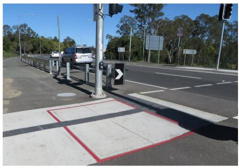
Figure 4.6(b) – Alternative outline red rectangular pavement marking
